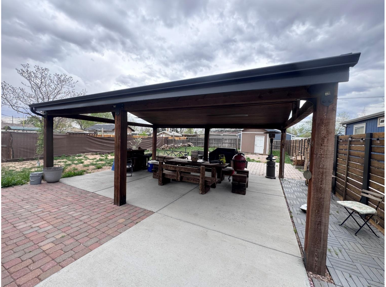
Photo of the subject shade structure facing south
