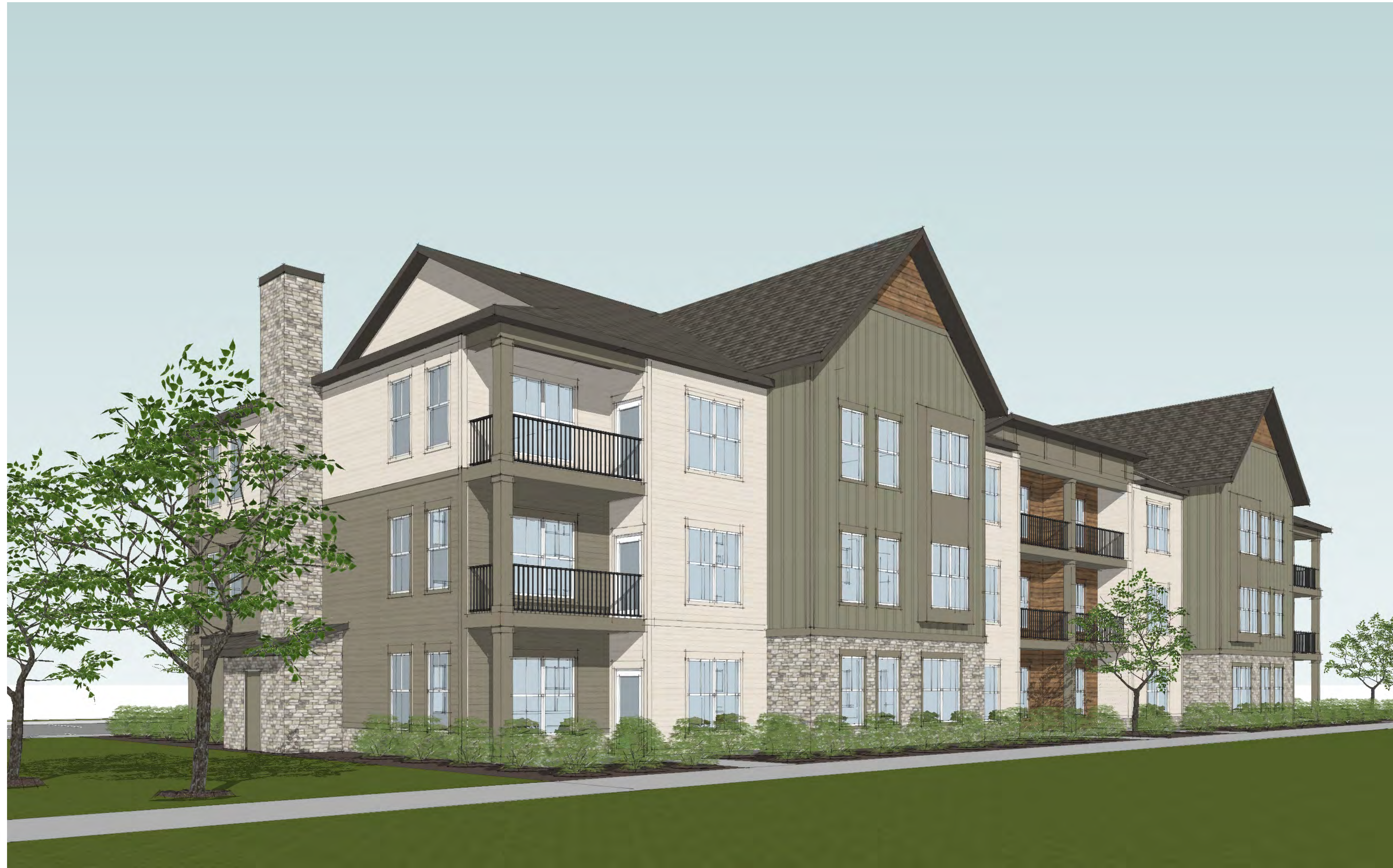
VIEW FROM STREET/COURTYARD LOOKING AT APARTMENT BUILDING TYPE D 3-STORY
