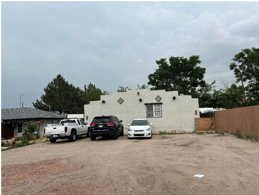
Existing two unit residential building (taken June 14, 2024)
