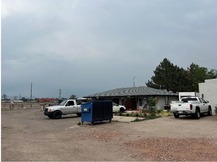
Existing four unit residential building (taken June 14, 2024)
