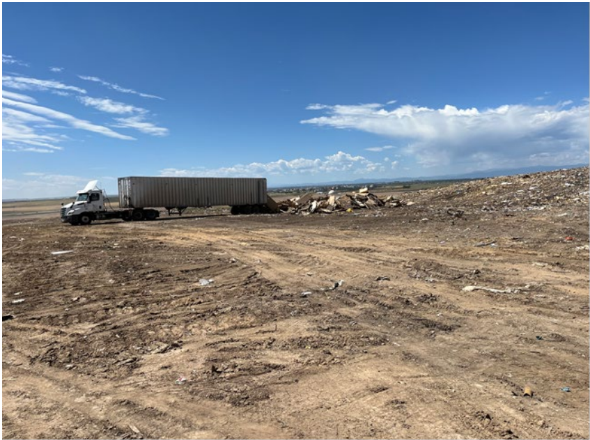
Picture 5: Construction and Demolition Debris Disposal Area Looking Southwest
