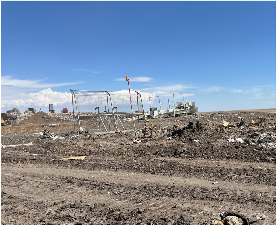
Picture 7: MSW Working Face Looking Northeast
