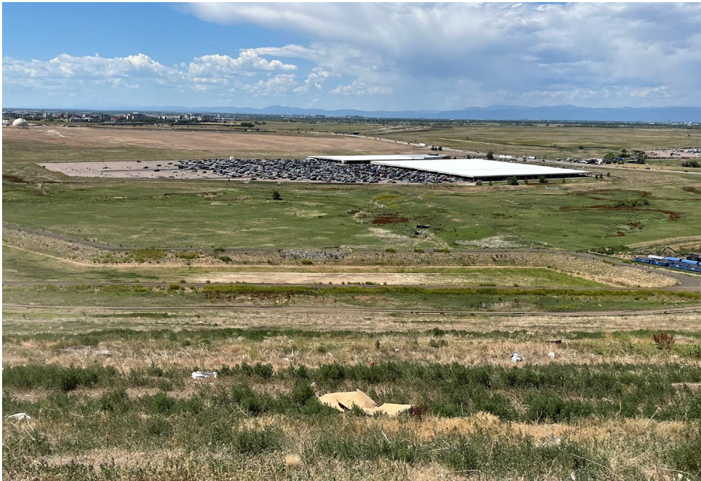
Picture 11: Retention Pond Totally Dry Looking Southwest
