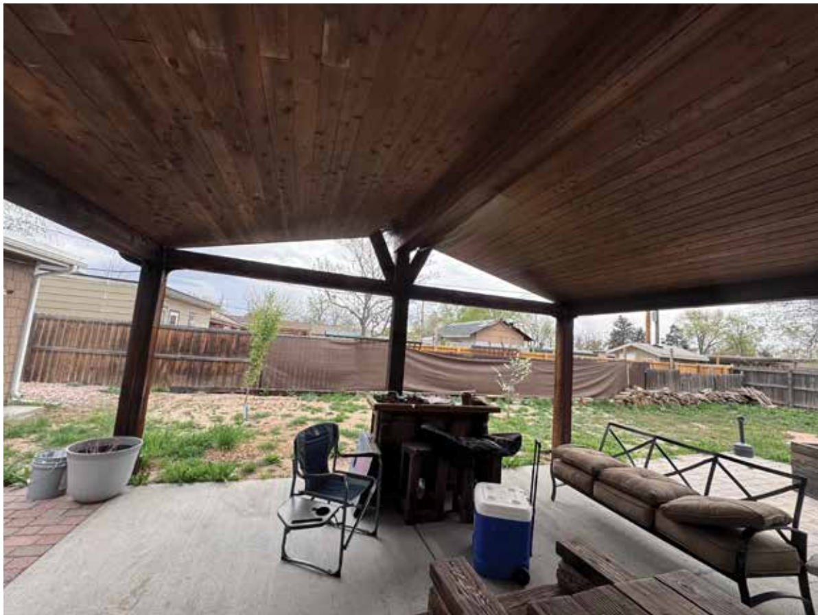
Within the structure facing east
