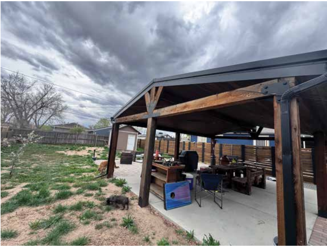
Facing southwest towards the structure
