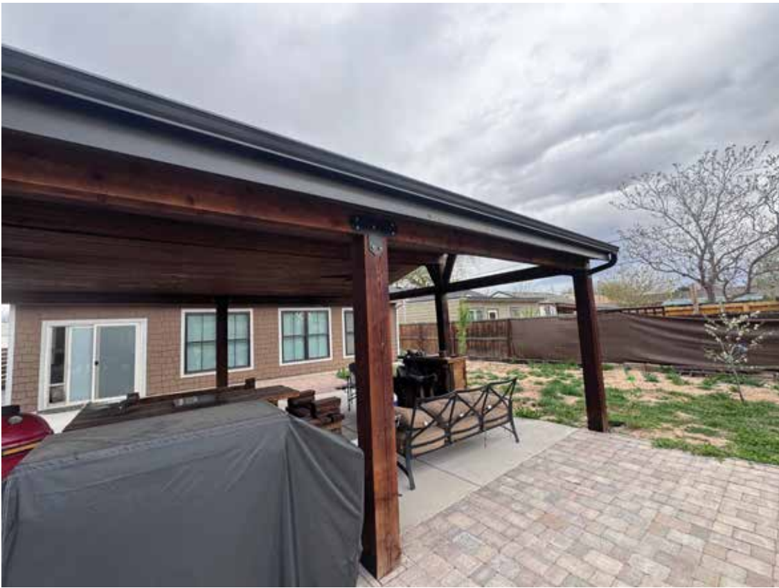
Facing northeast towards the structure
