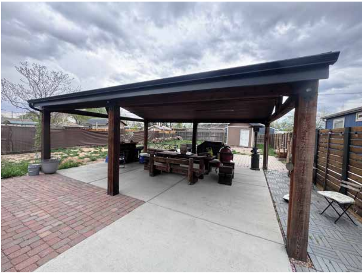
Facing south towards the structure
