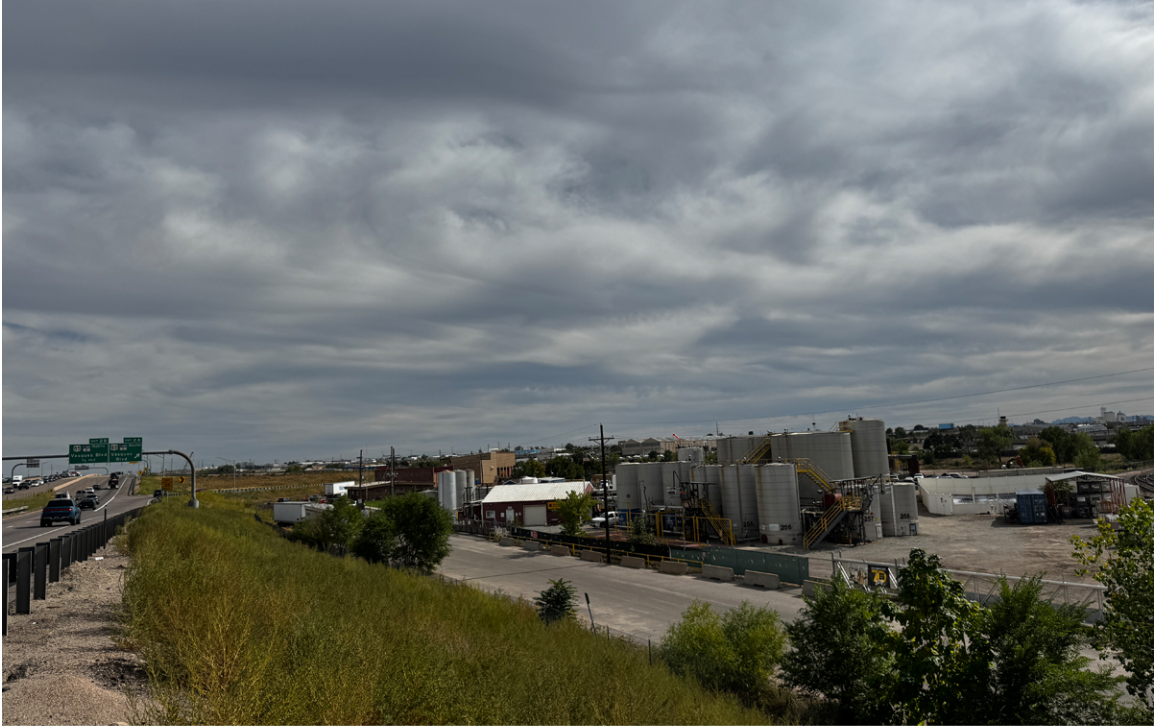
Existing View from the Northwest
