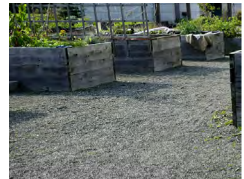
CRUSHER FINES PATH
