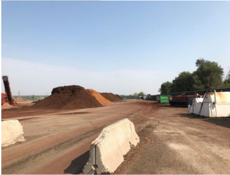
Water trucks for dust mitigation and internal access roads free of obstruction and trash
