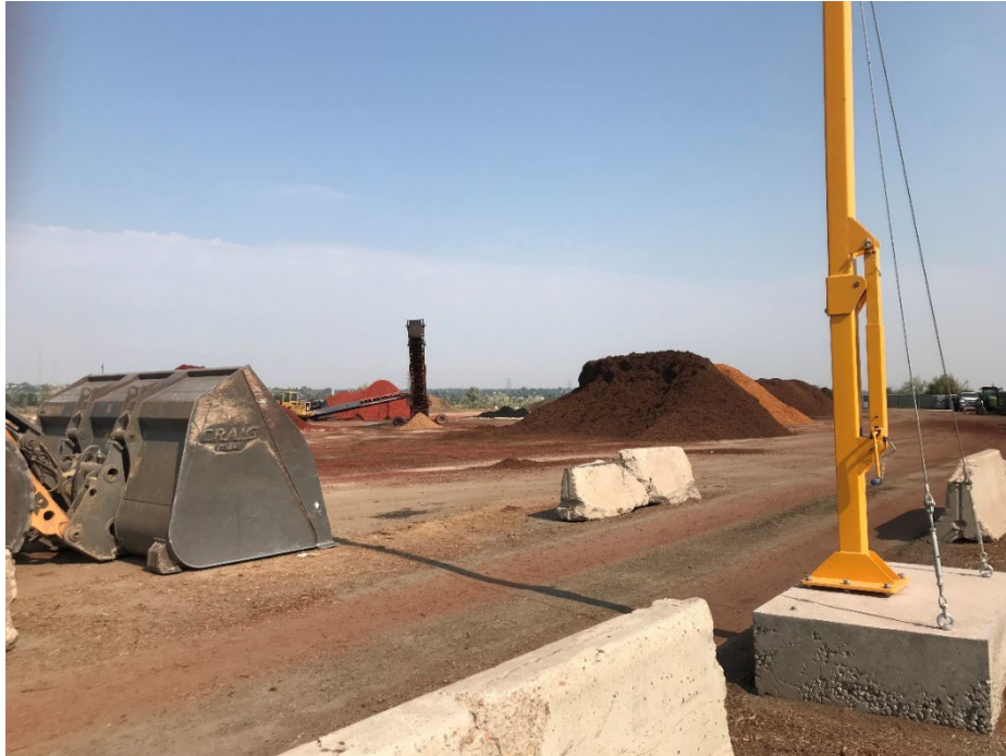
Exhibit D Premises kept free of garbage, trash, and excessive debris at all times. Depiction showing recycled asphalt internal roads
