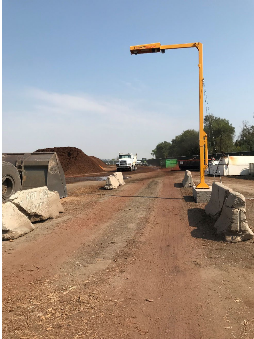
Image depicting Dust Mitigation – Water Truck and showing recycled asphalt road base
