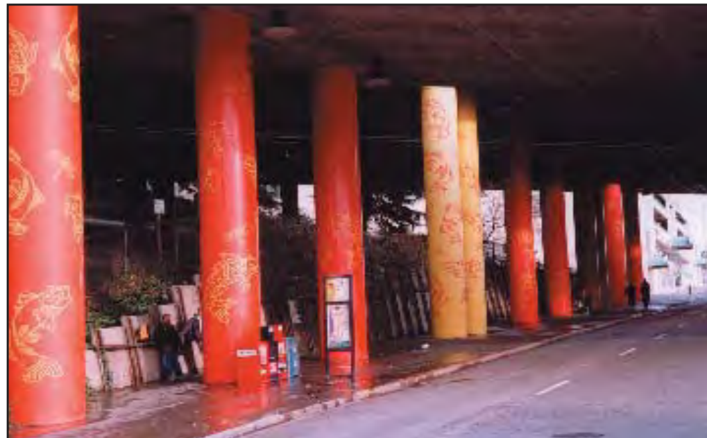
Painted colonnades underneath the I-5 freeway
