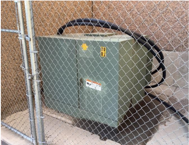
Exterior Transformer – Locked gate and oil leakage
