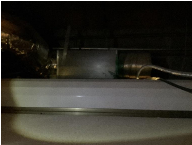
Carrier Bladder Air Terminal Unit (Abandoned)
