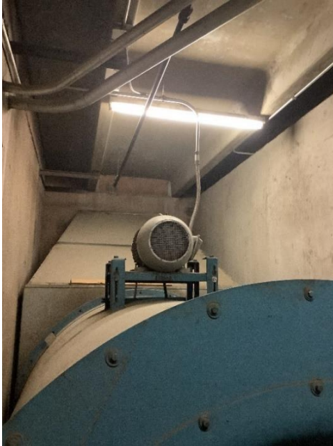
Building Exhaust Fan (EF)-1
