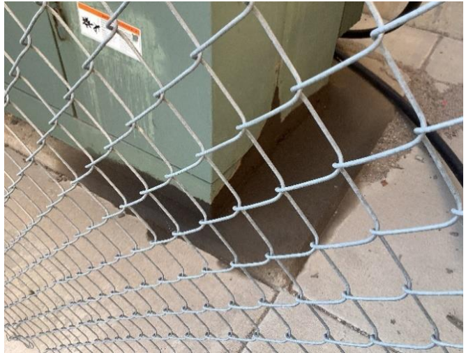
Exterior Transformer – oil leakage
