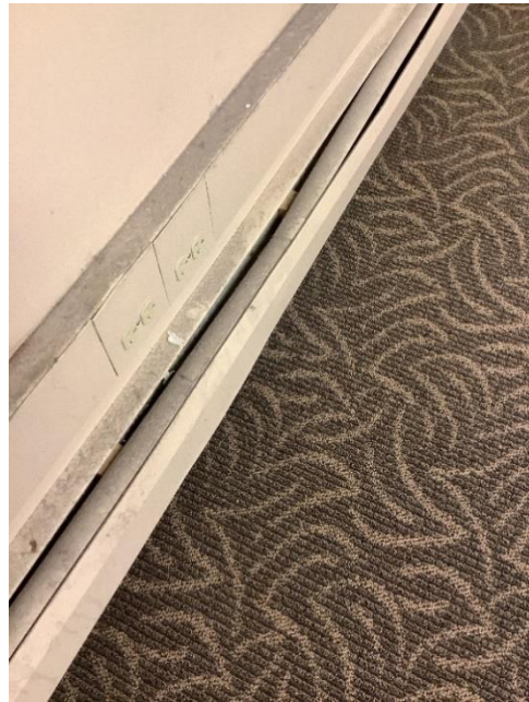
HW Baseboard Units – damage and deformation
