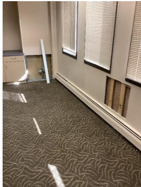
South Suite Conference Room - drywall water damage repair in progress
