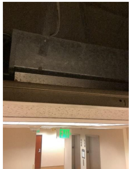
Carrier Bladder Air Terminal Unit (Abandoned)
