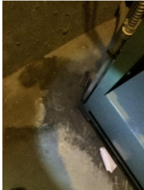
Loading Dock elevator – Leakage at motor gearbox
