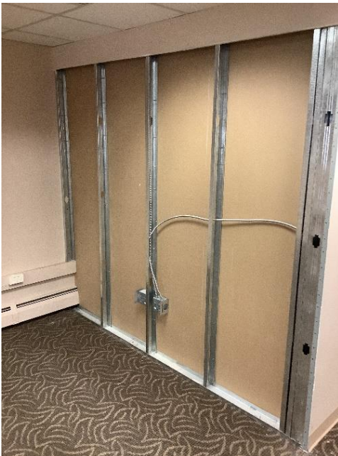
North Suite - office drywall water damage repair in progress
