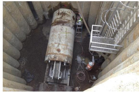
Example of trenchless construction method. Photo source: HDR
