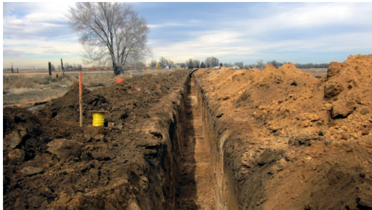
Trench for sub-surface produced water pipeline in Weld County Source: Colorado Public Radio, photo by Lesley McClurg, 2014
