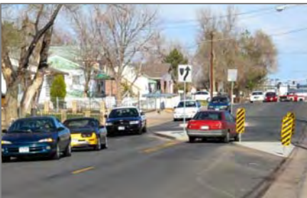
Traffic calming at East 60 th Avenue and Olive Street. (Photo: FHU)
