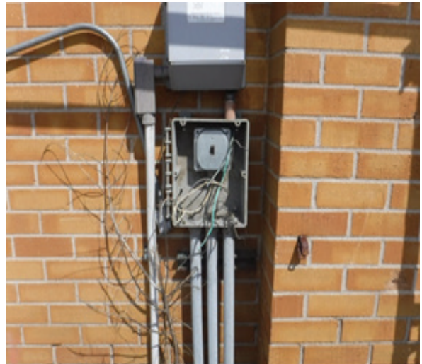
Exposed Wires
