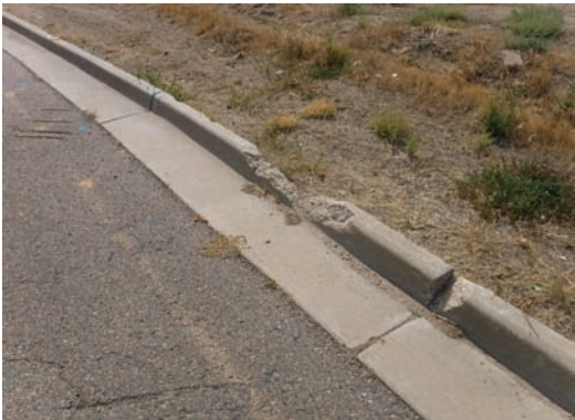
Deteriorated Curb/Sidewalk
