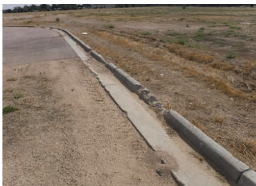
Deteriorated Curb/Sidewalk
