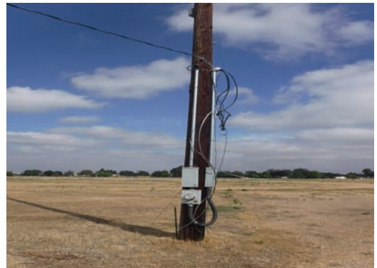
Deteriorated Electrical Pole
