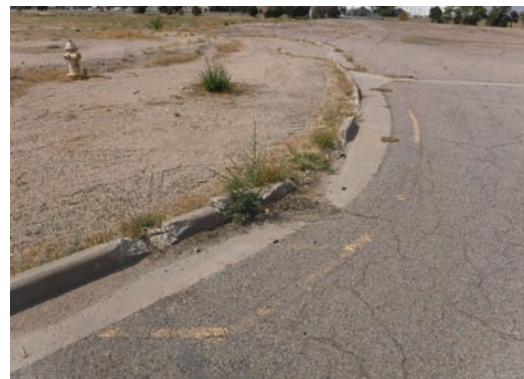
Deteriorated Curb/Sidewalk
