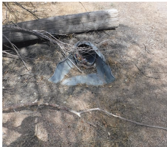
Deteriorated Stormwater Improvements
