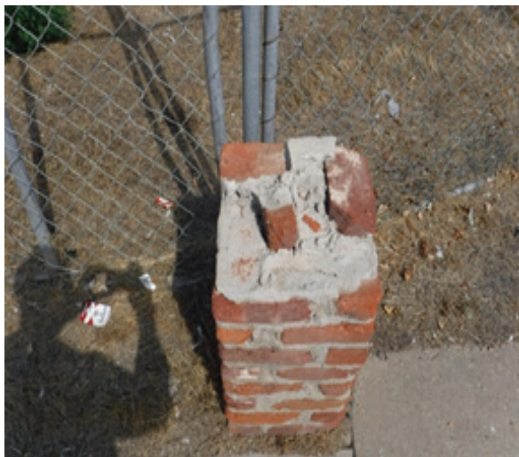
Deteriorated Support Post
