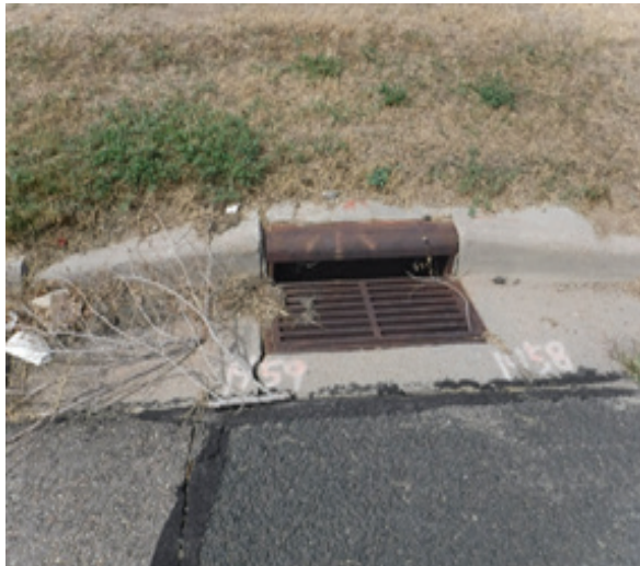
Deteriorated Stormwater Systems
