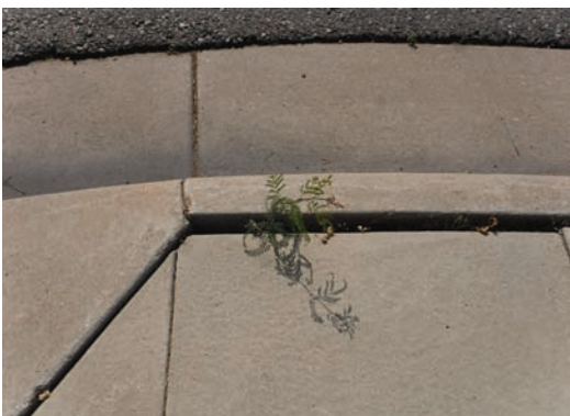
Cracked/Uneven Pedestrian Surfaces
