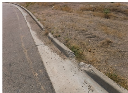
Deteriorated Curb/Sidewalk
