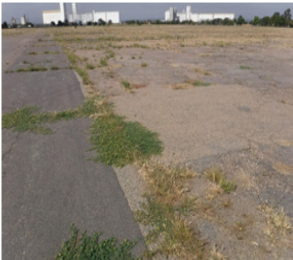
Deteriorated Paving
