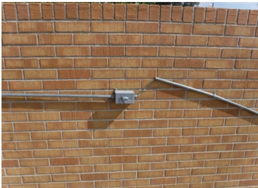
Unsafe/Exposed Electrical Wire
