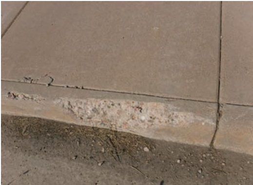
Deteriorated Curb/Sidewalk
