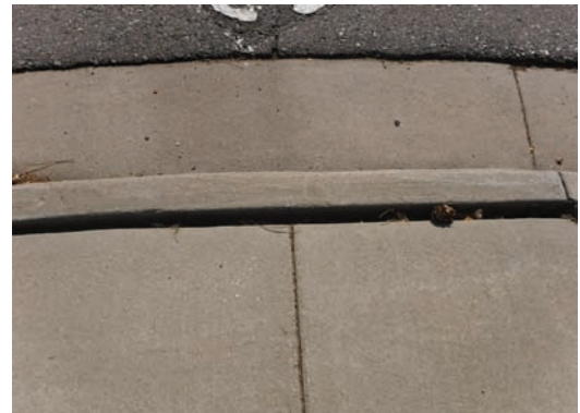
Cracked/Uneven Pedestrian Surfaces
