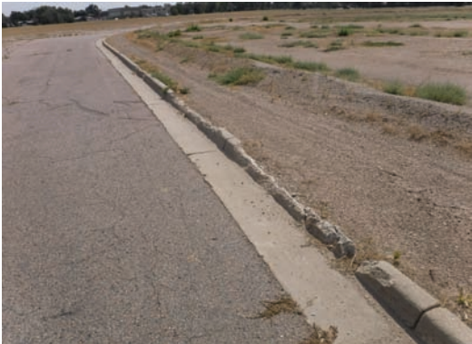
Deteriorated Curb/Sidewalk
