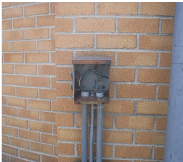
Unsafe/Exposed Electrical Wire
