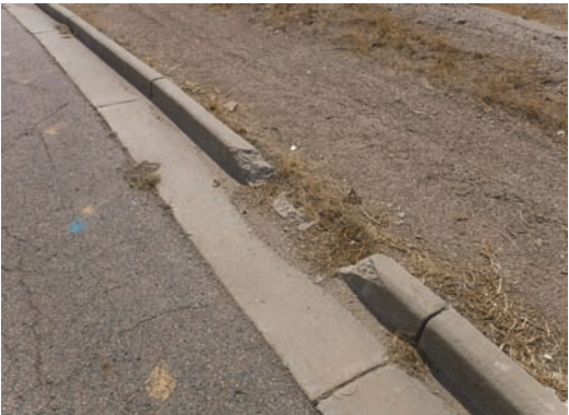
Deteriorated Curb/Sidewalk
