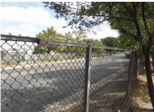
Dilapidated/Deteriorated Fencing
