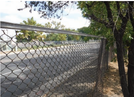
Dilapidated/Deteriorated Fencing
