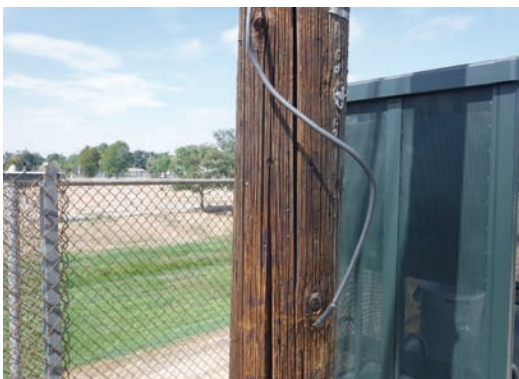
Unsafe/Exposed Electrical Wire
