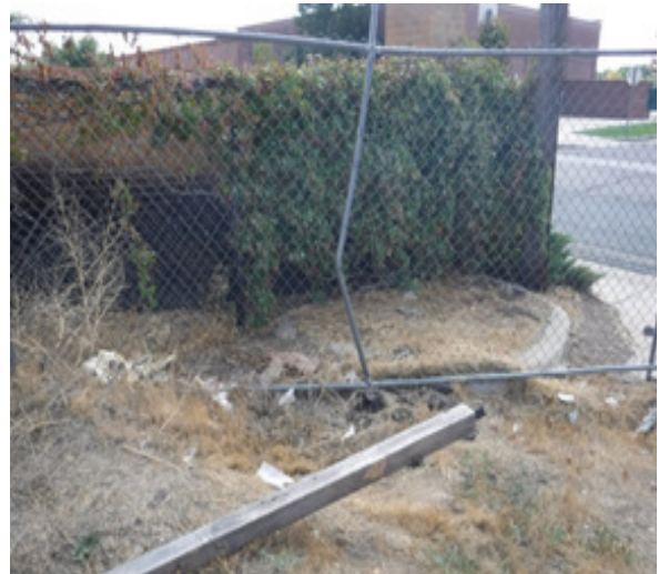
Bent/Broken Fence
