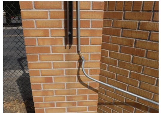
Unsafe/Exposed Electrical Wire
