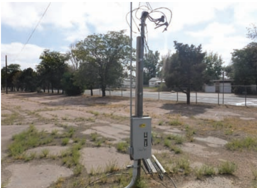
Deteriorated Electrical Pole
