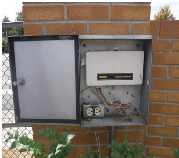
Unsafe/Exposed Electrical Wire
