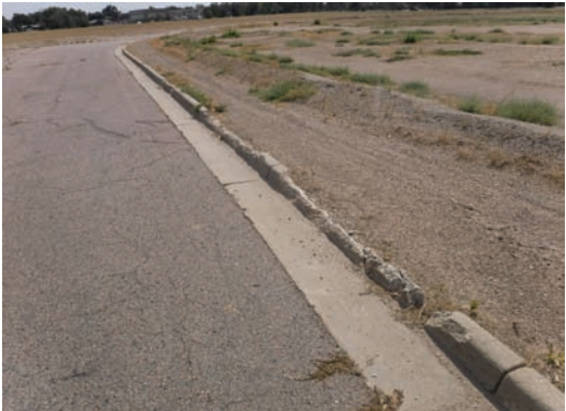
Deteriorated Curb/Sidewalk
