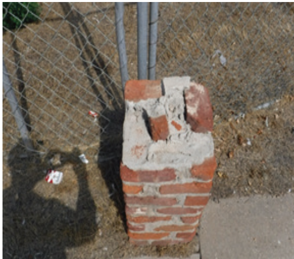
Deteriorated Support Post
