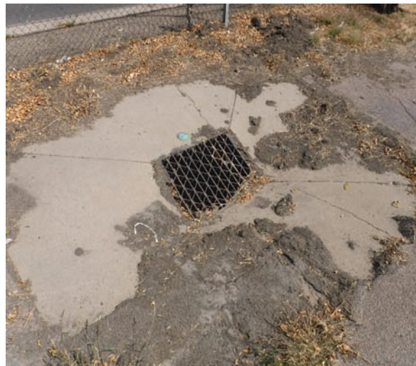
Deteriorated Stormwater Improvements
