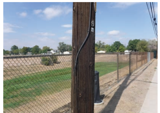
Unsafe/Exposed Electrical Wire
