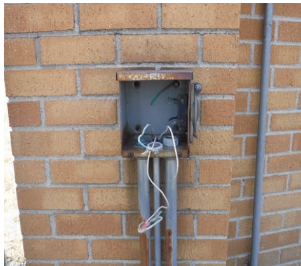
Unsafe/Exposed Electrical Wire
