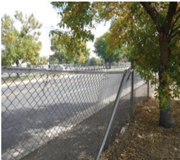
Bent/Broken Fence
