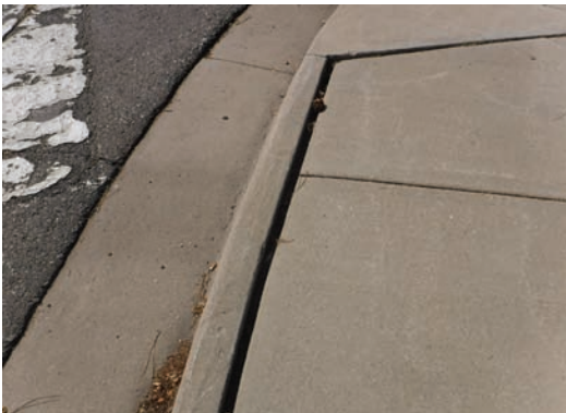
Cracked/Uneven Pedestrian Surfaces
