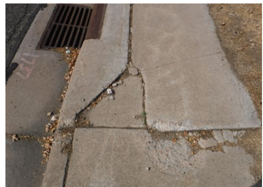
Cracked/Uneven Pedestrian Surfaces
