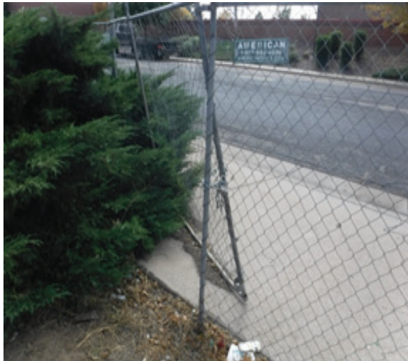
Bent/Broken Fence
