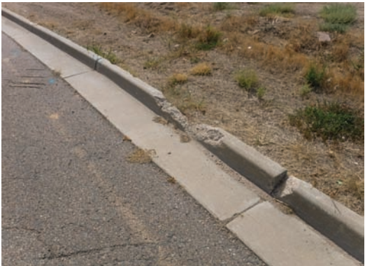
Deteriorated Curb/Sidewalk
