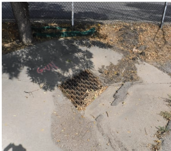
Deteriorated Stormwater Improvements
