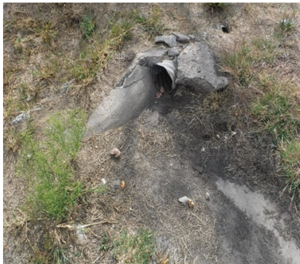
Deteriorated Stormwater Improvements
