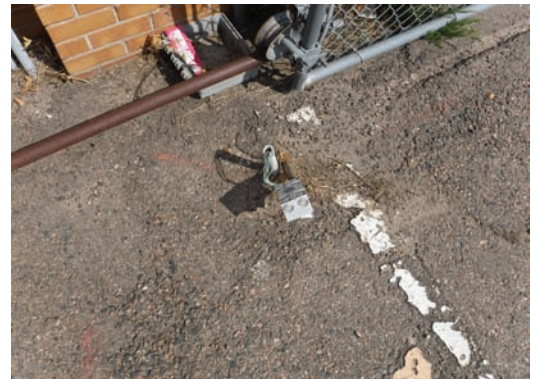
Unsafe/Exposed Electrical Wire
