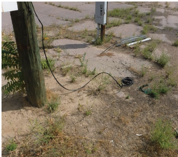
Unsafe/Exposed Electrical Wire
