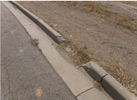
Deteriorated Curb/Sidewalk
