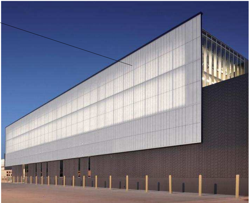
Translucent Fiberglass Wall Panel System example
