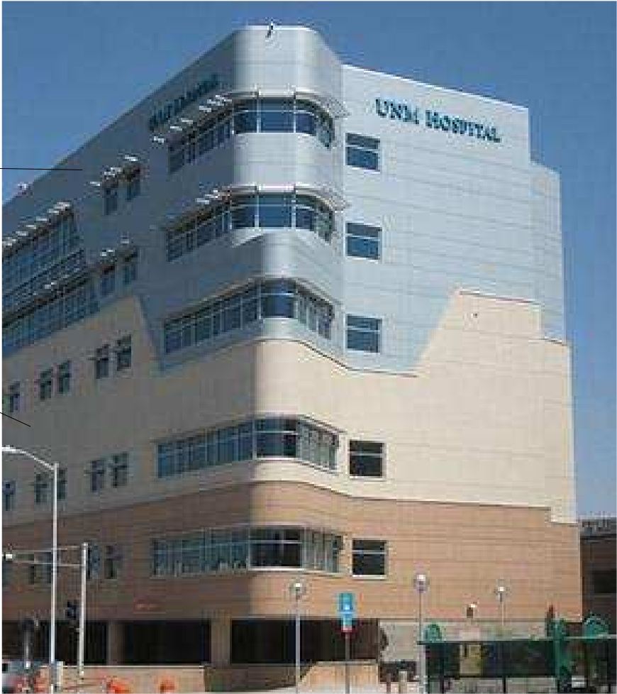
Cast in Place Concrete Wall with Exterior Insulation Finish System (EFIS) example
