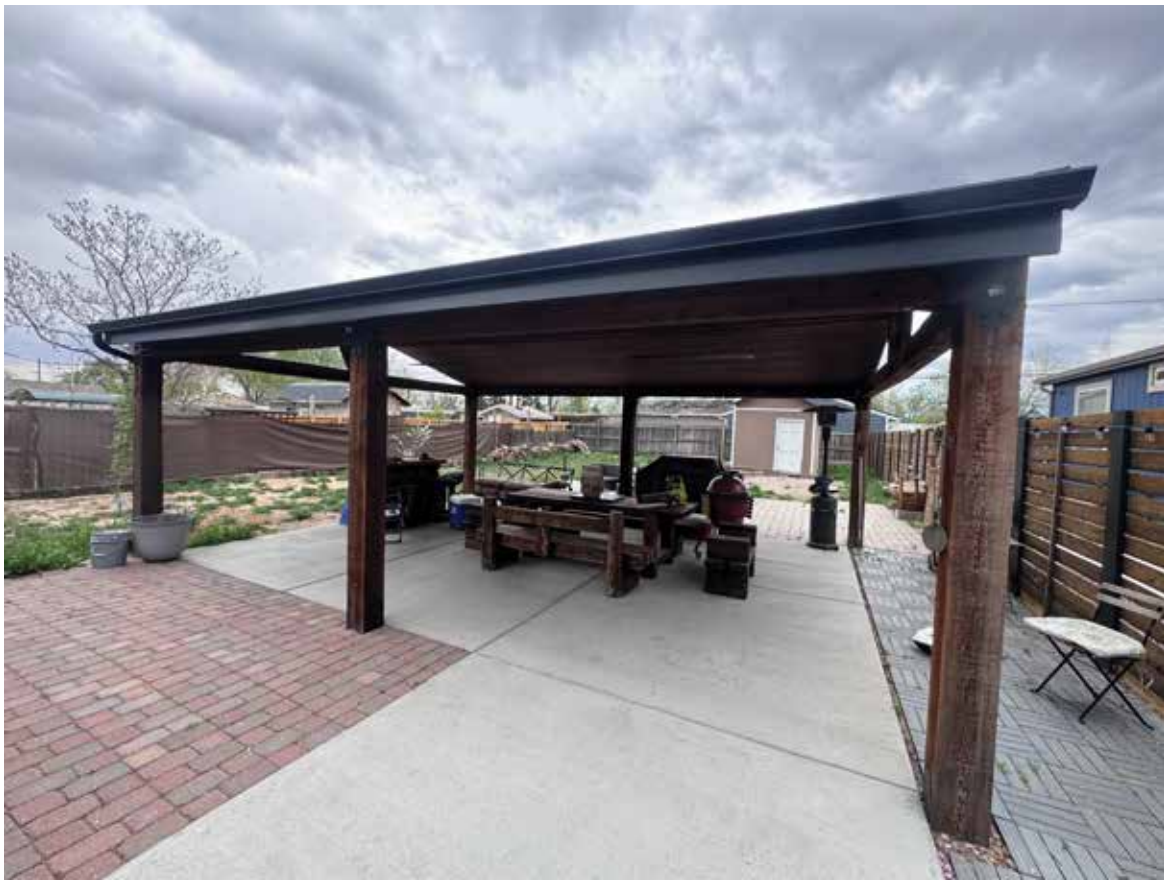
Facing south towards the structure
