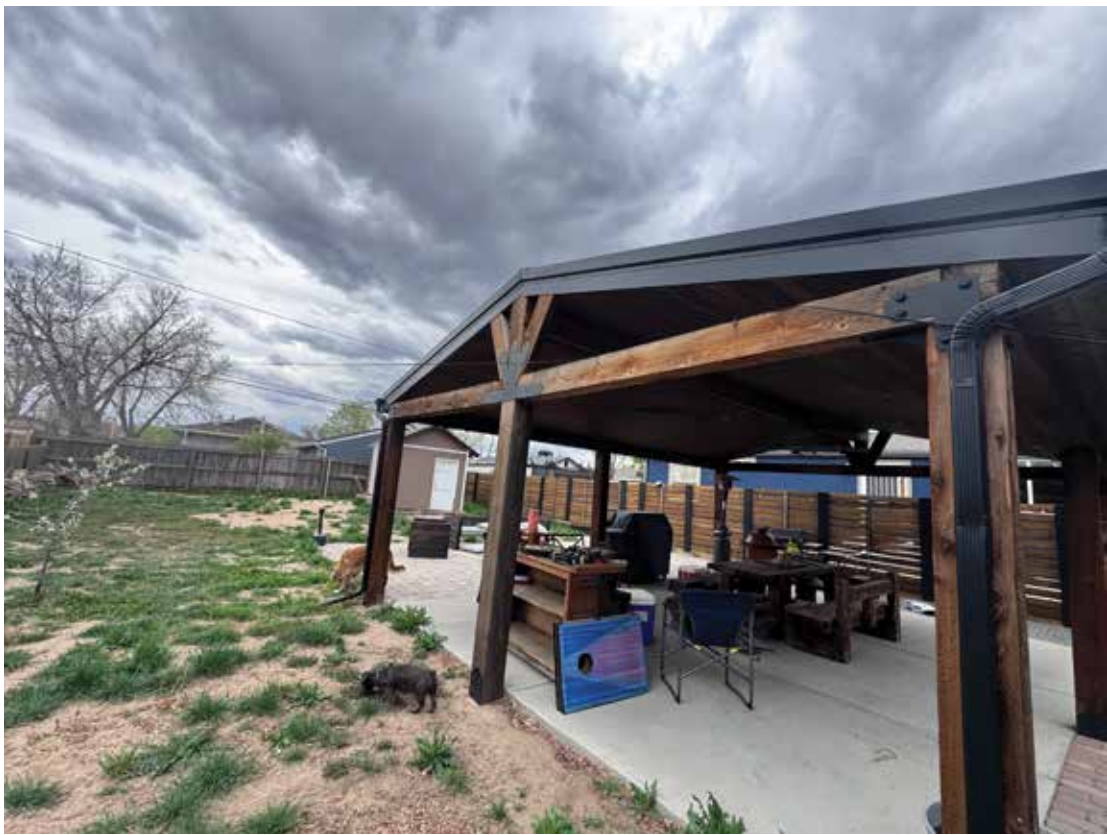
Facing southwest towards the structure
