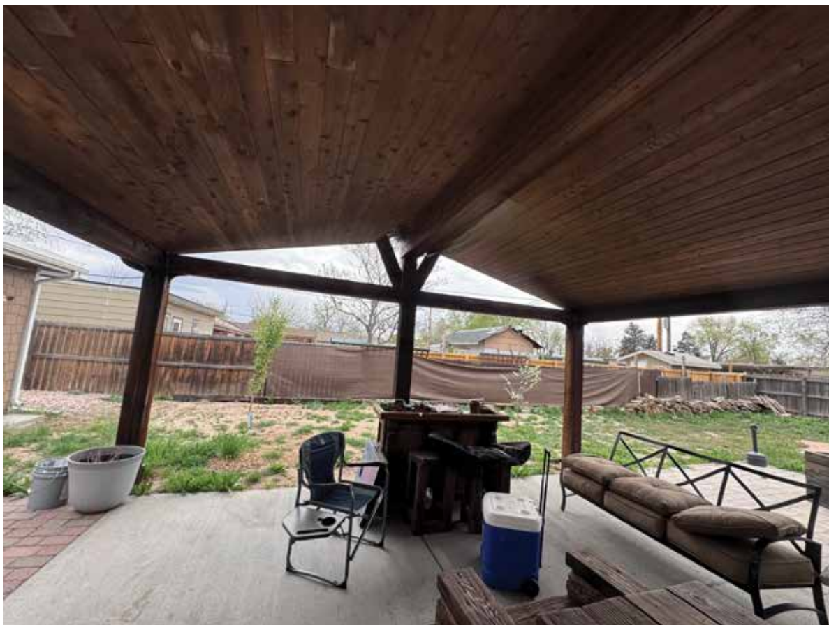
Within the structure facing east
