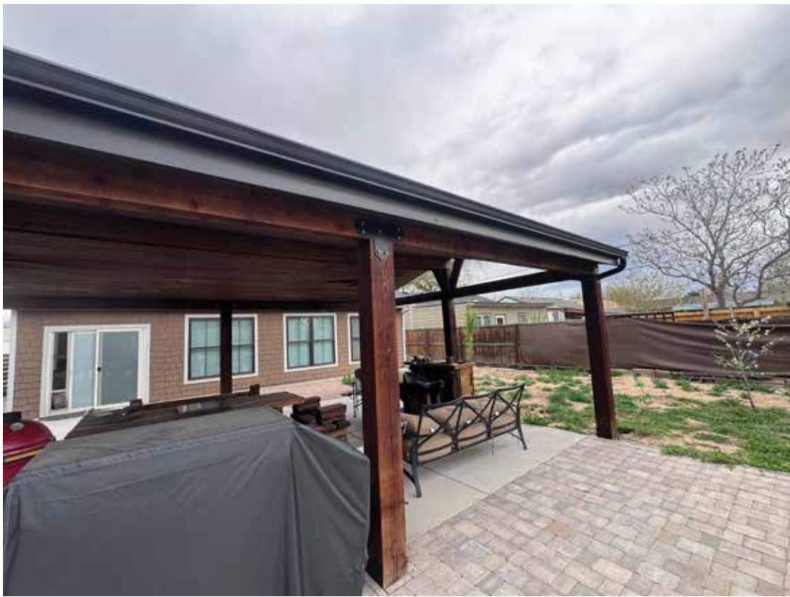
Facing northeast towards the structure
