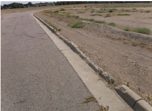
Deteriorated Curb/Sidewalk
