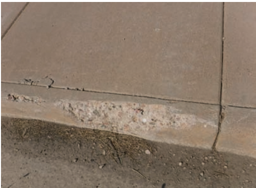
Deteriorated Curb/Sidewalk
