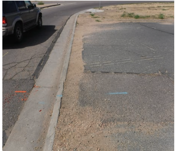
Lack of Access to Dahlia Street right-of-way
