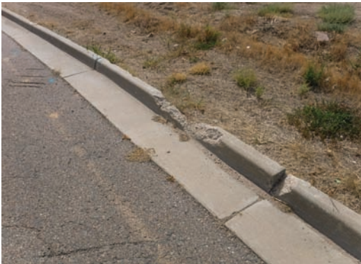
Deteriorated Curb/Sidewalk
