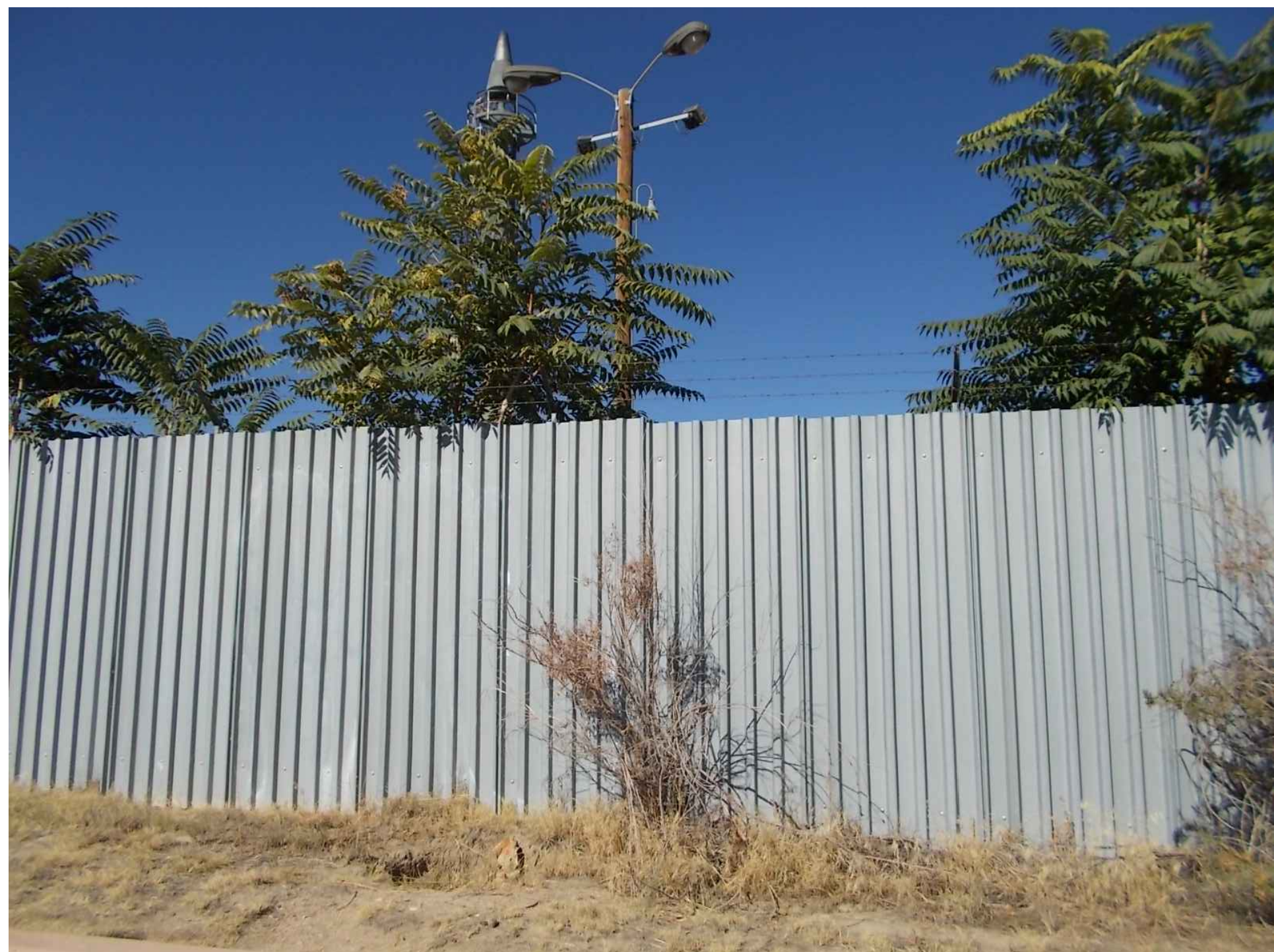
MUELLER METAL SCREEN WALL (8' TALL) (OR APPROVED EQUAL) (INSTALL 3 STRAND BARB WIRE ALONG THE TOP OF THE SCREEN WALL)
