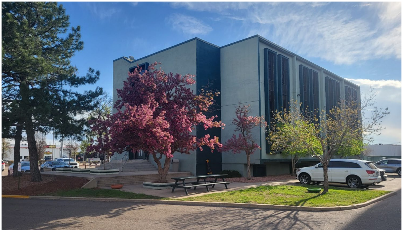
Stout Street's adminstration Building from the east along the Sand Creek Trail
