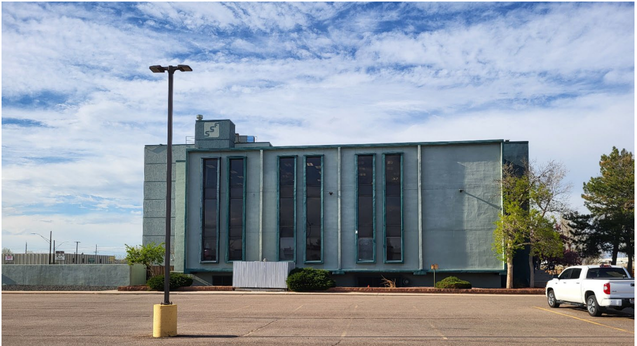
Stout Street's adminstration Building from the South along East 49 th Avenue
