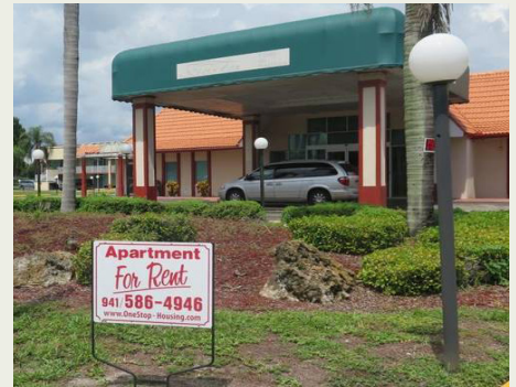
The Knights Inn in Bradenton, Fla., was converted to affordable apartments. Apartments cost ~$625 per month, which includes utilities.
