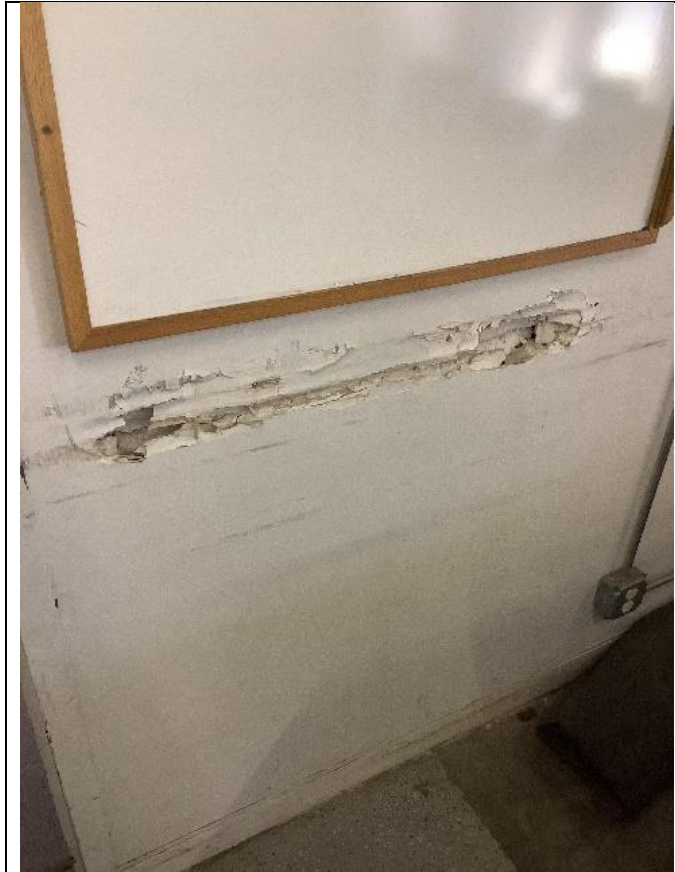
Damaged drywall
