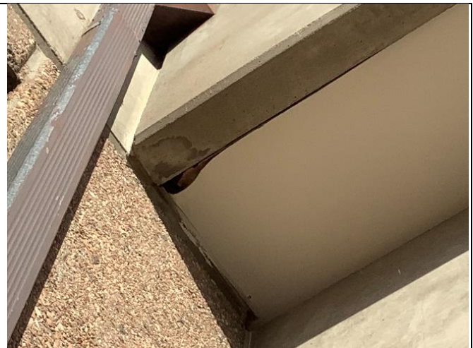
Water-damaged soffits
