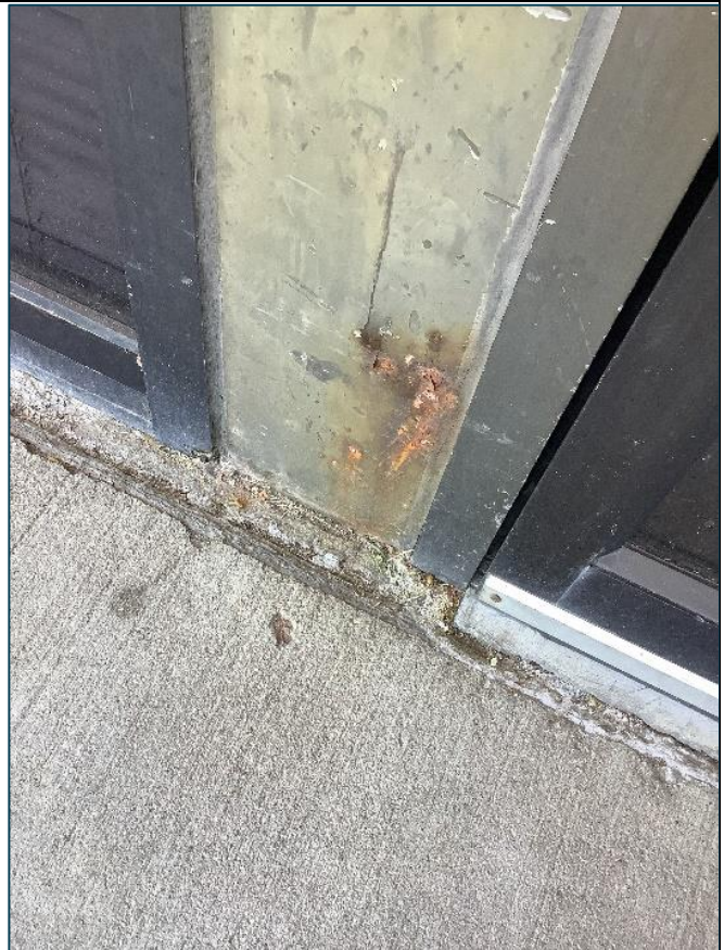
Localized corrosion adjacent to door frame
