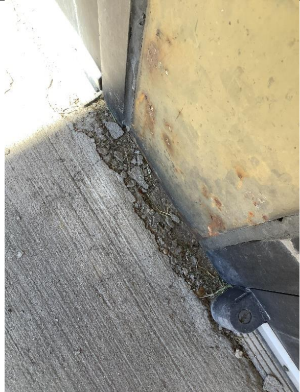
Localized sidewalk damage
