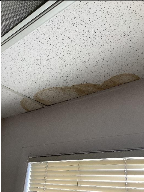
Water-stained ceiling tiles
