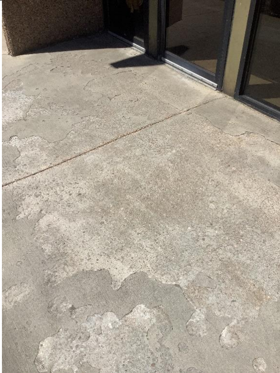
Localized surface spalling due to salt
