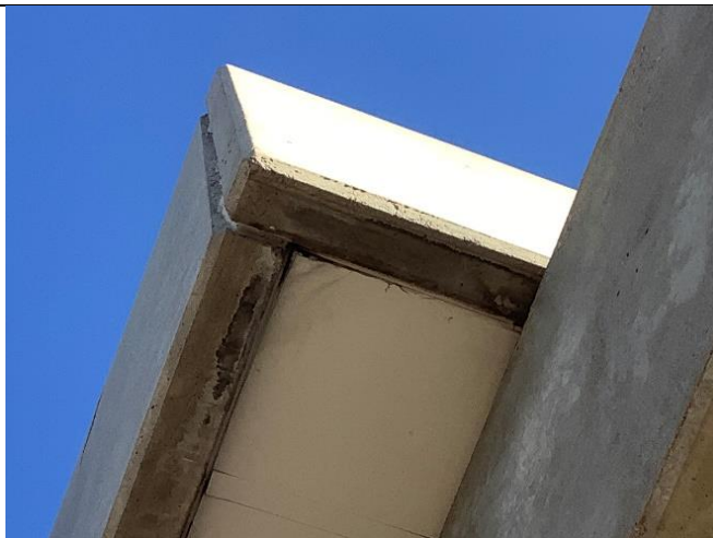
Water-damaged soffits
