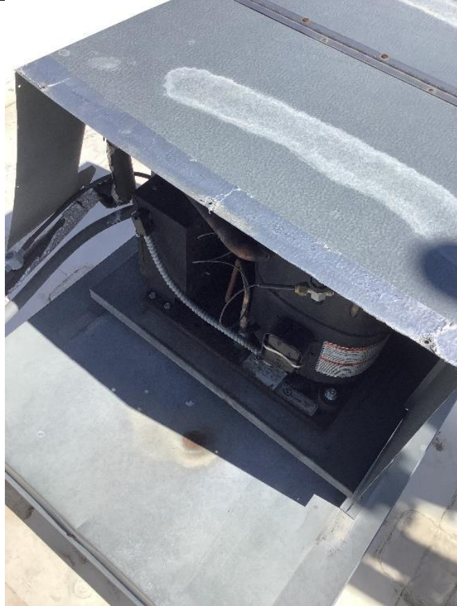
Missing panels on condensing unit
