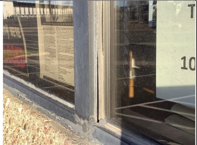
Localized seal failure
