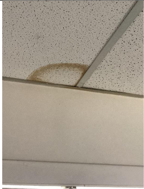
Water-stained ceiling tiles
