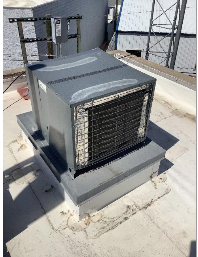
Condenser coil held in place with metallic tape
