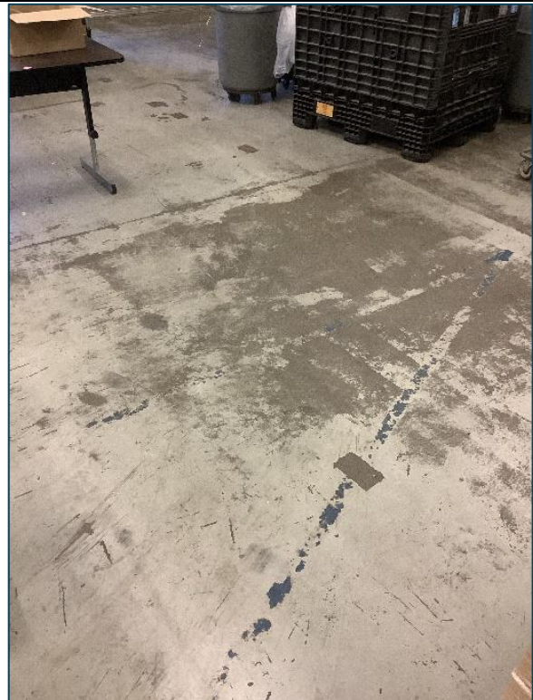
Surface finish wear on concrete floor
