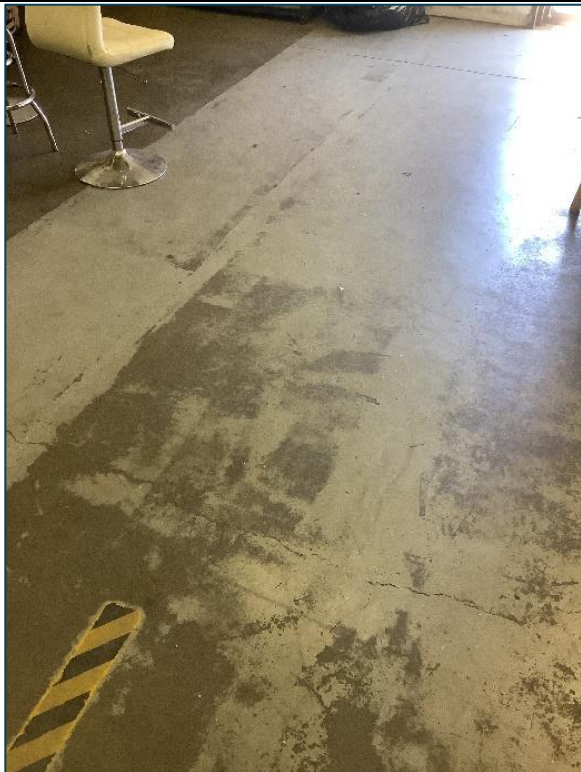
Minor cracking in concrete floors
