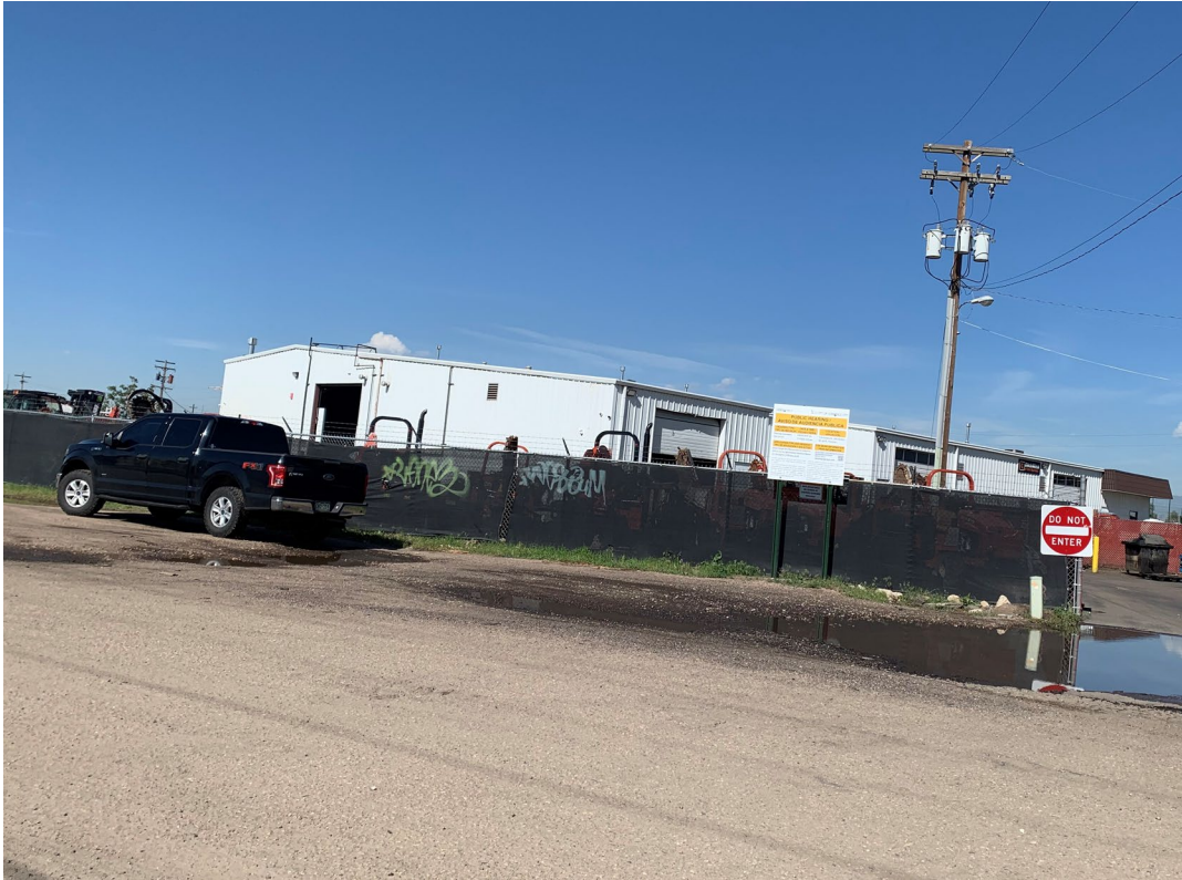
View from Elm Street (Taken May 30, 2023)
