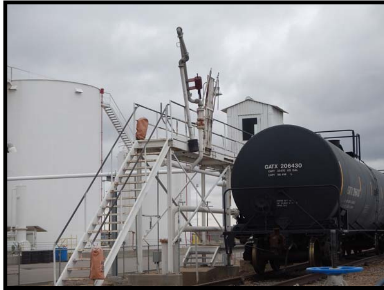
Figure 16: Existing Top-Loading Location of Rail Cars
