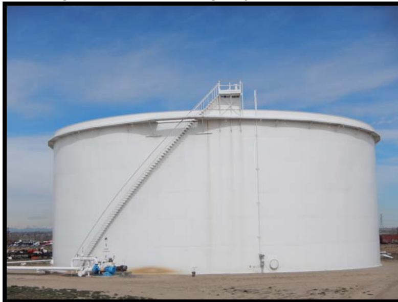
Figure 3: External Floating Roof – Tank #12
