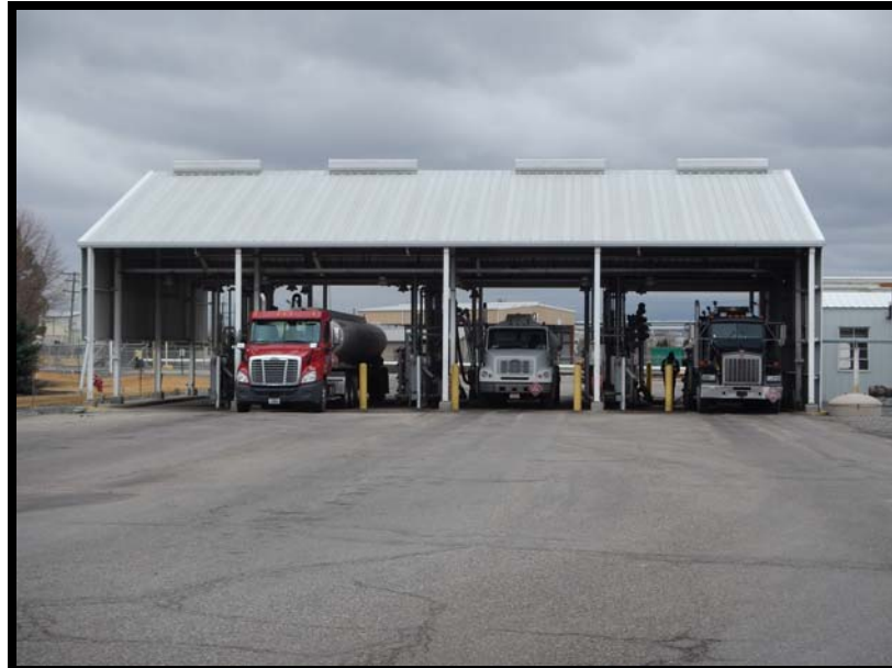
Figure 11: Existing Truck Loading / Unloading Canopy (3-Bay)
