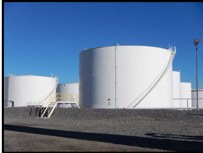
Figure 6: Existing Earthen Diked Containment
