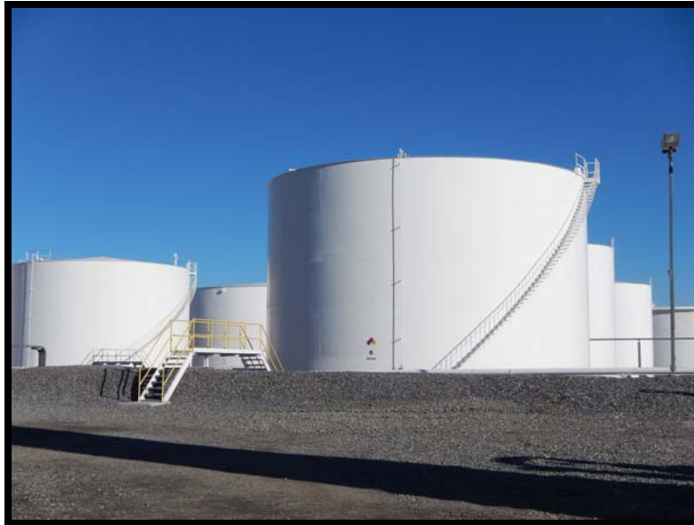
Figure 4: Fixed Cone Roof – Tank #6
