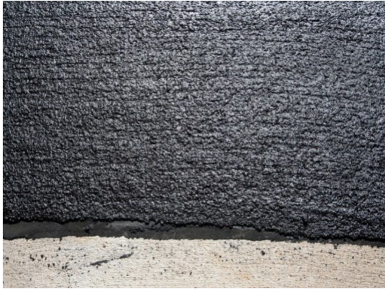
Slurry Seal Application
