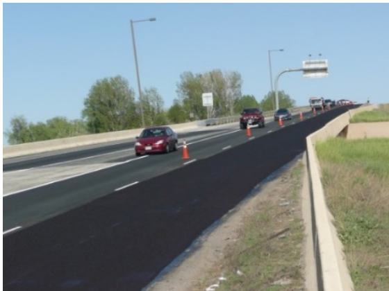
Micro surfacing Application
