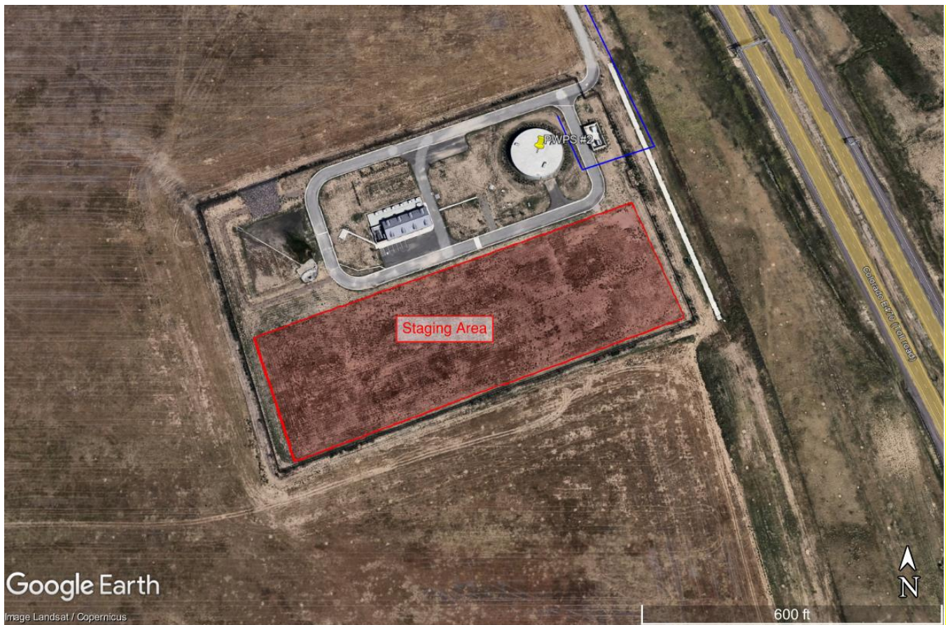
Figure 6-1: Construction Staging Area
