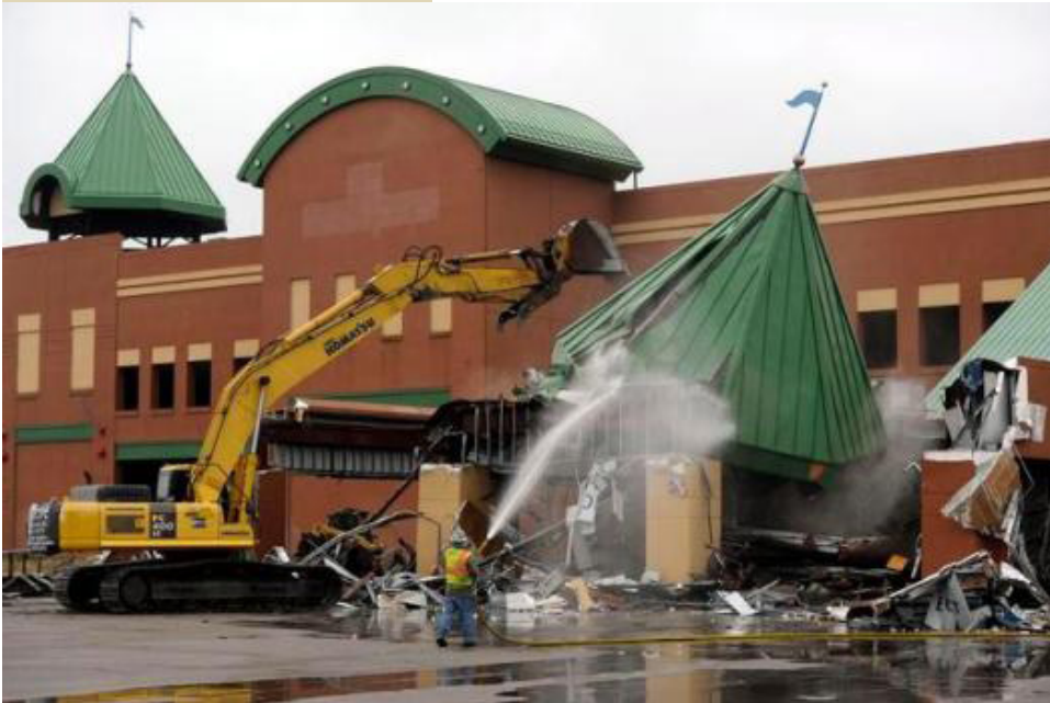
Mile High Greyhound Park demolition
