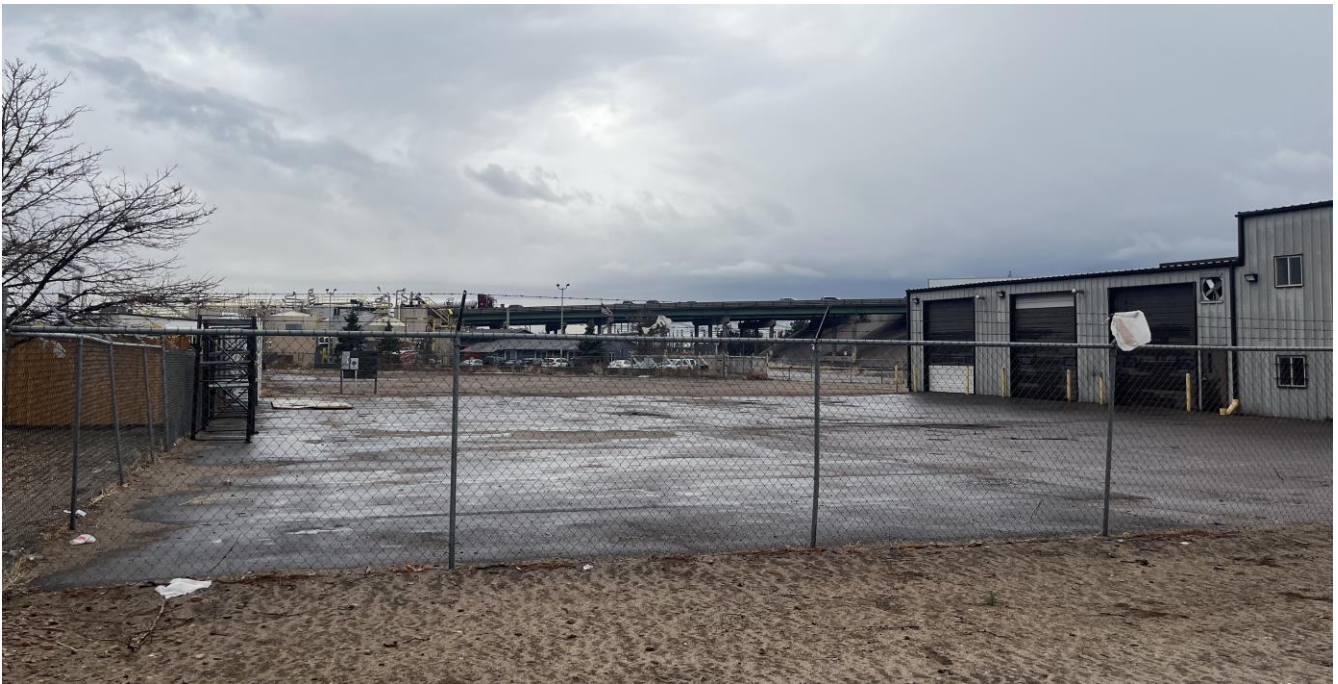
View of the property from 60 th Avenue facing south
