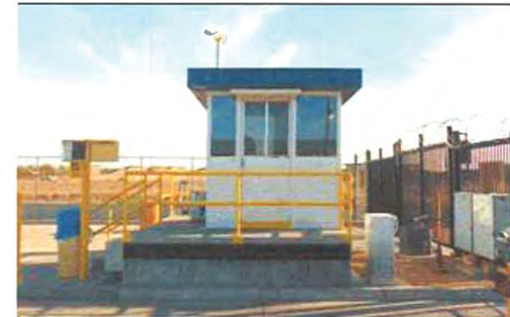
West view of the inspection booth
