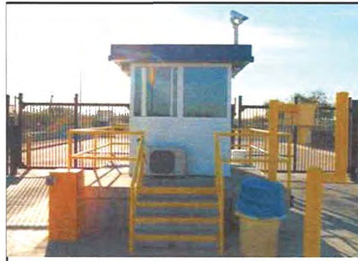
Rear view of the inspection booth
