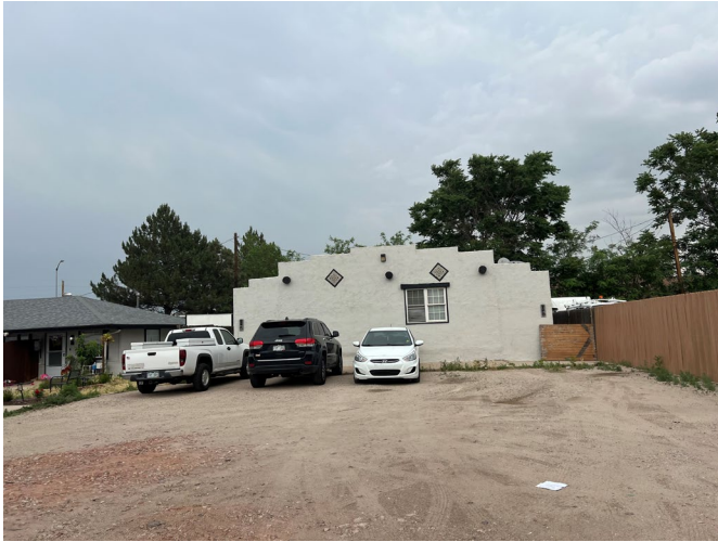
Existing two unit residential building (taken June 14, 2024)
