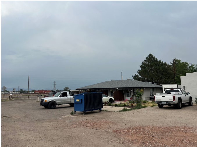
Existing four unit residential building (taken June 14, 2024)
