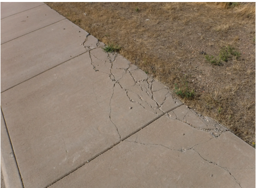
Deteriorated Curb/Sidewalk
