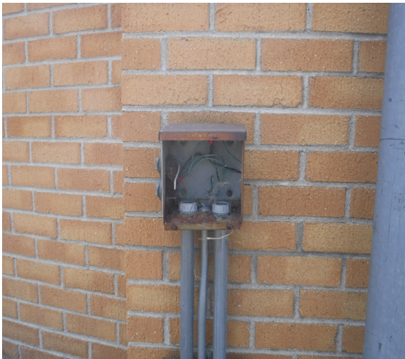
Unsafe/Exposed Electrical Wire
