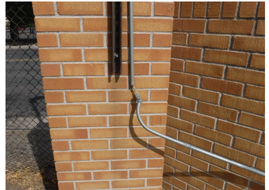
Unsafe/Exposed Electrical Wire
