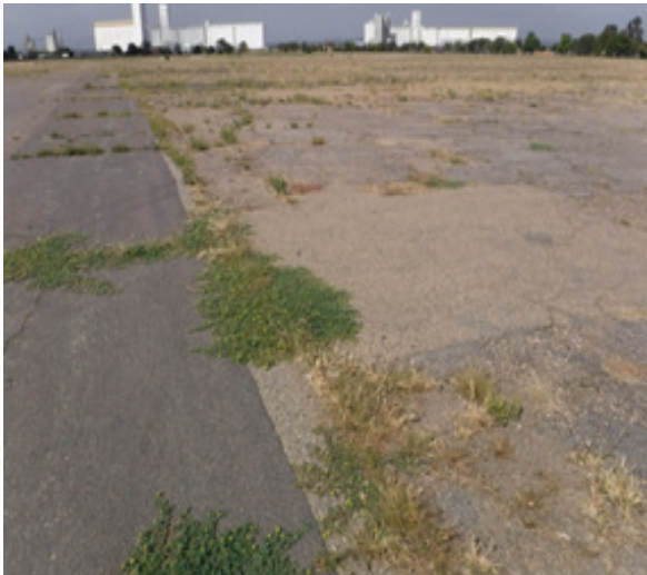
Deteriorated Paving
