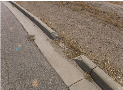
Deteriorated Curb/Sidewalk
