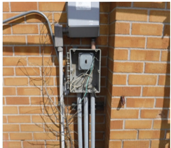
Exposed Wires
