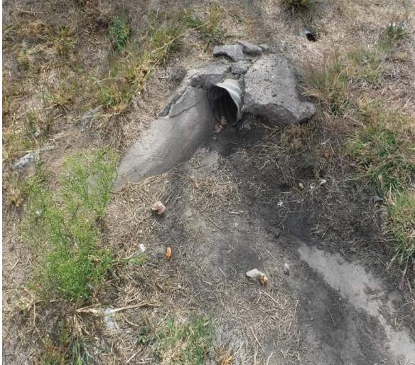
Deteriorated Stormwater Improvements
