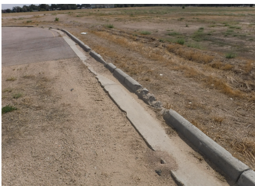
Deteriorated Curb/Sidewalk
