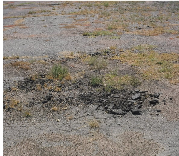
Deteriorated Paving
