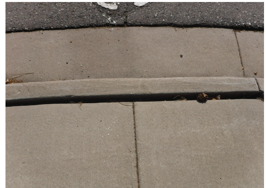
Cracked/Uneven Pedestrian Surfaces
