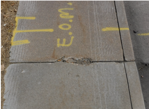
Cracked/Uneven Pedestrian Surfaces
