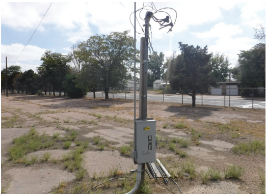
Deteriorated Electrical Pole
