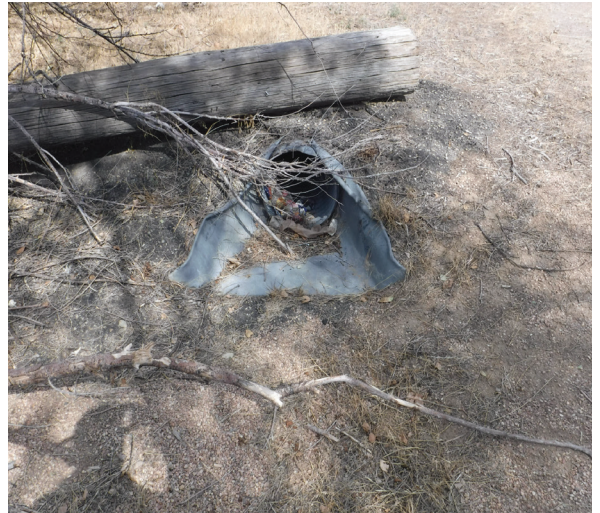
Deteriorated Stormwater Improvements
