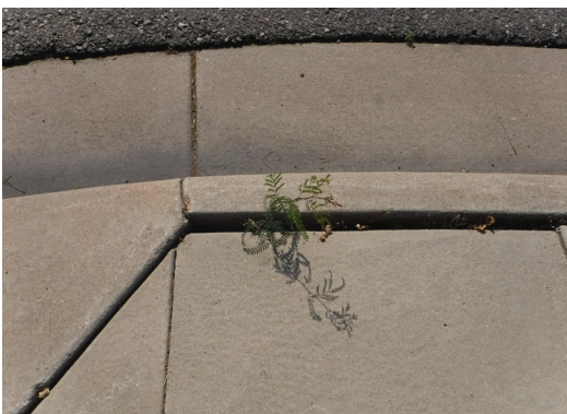
Cracked/Uneven Pedestrian Surfaces
