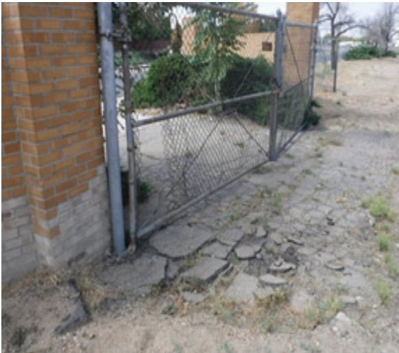
Unsafe Paving
