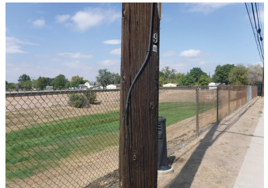
Unsafe/Exposed Electrical Wire
