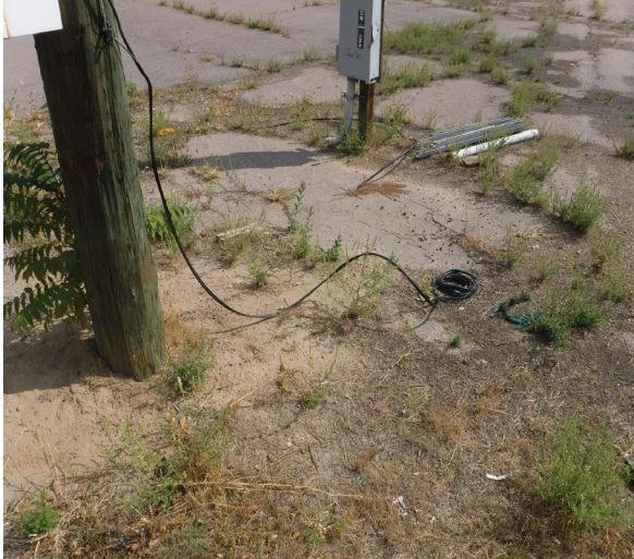
Unsafe/Exposed Electrical Wire
