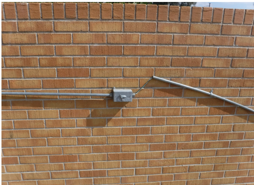
Unsafe/Exposed Electrical Wire
