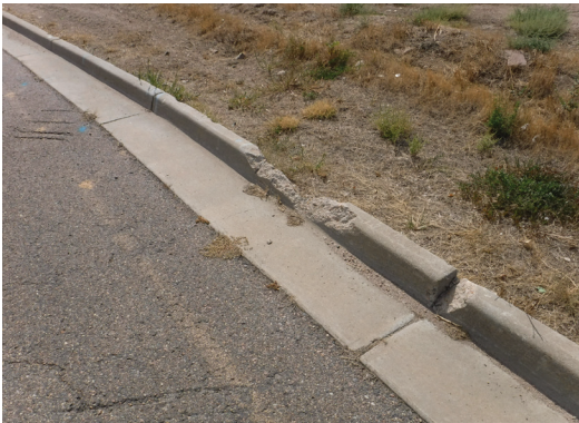
Deteriorated Curb/Sidewalk
