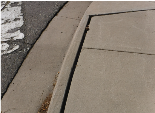
Cracked/Uneven Pedestrian Surfaces
