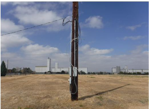
Deteriorated Electrical Pole
