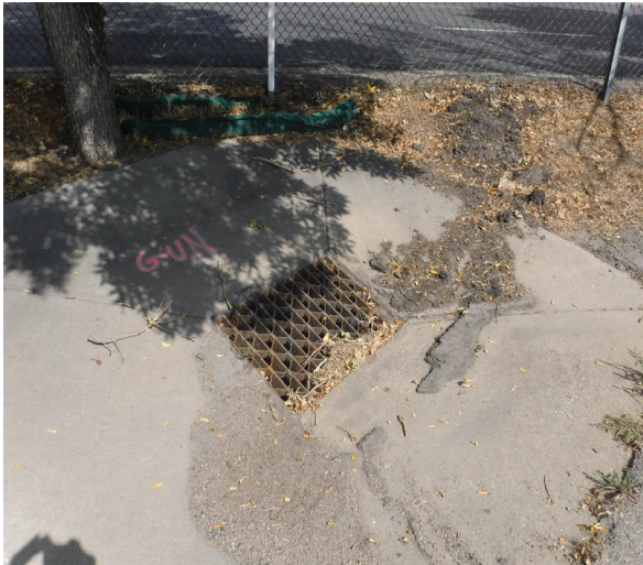
Deteriorated Stormwater Improvements
