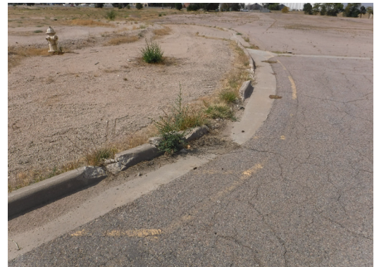
Deteriorated Curb/Sidewalk
