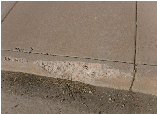
Deteriorated Curb/Sidewalk
