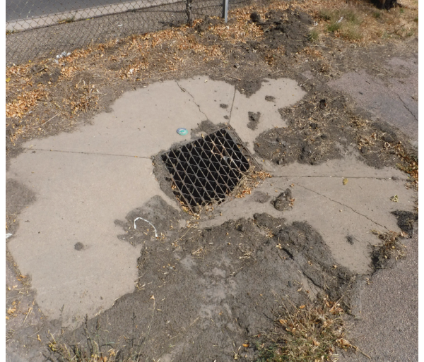
Deteriorated Stormwater Improvements
