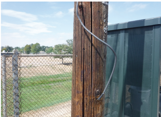
Unsafe/Exposed Electrical Wire
