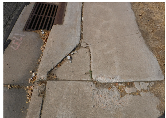
Cracked/Uneven Pedestrian Surfaces
