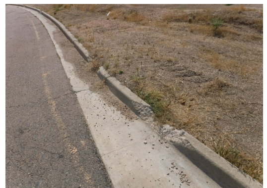
Deteriorated Curb/Sidewalk
