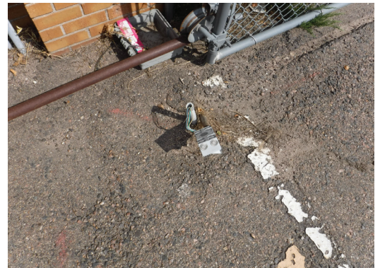
Unsafe/Exposed Electrical Wire
