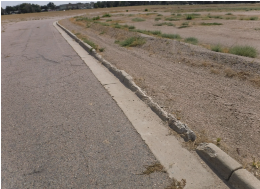
Deteriorated Curb/Sidewalk
