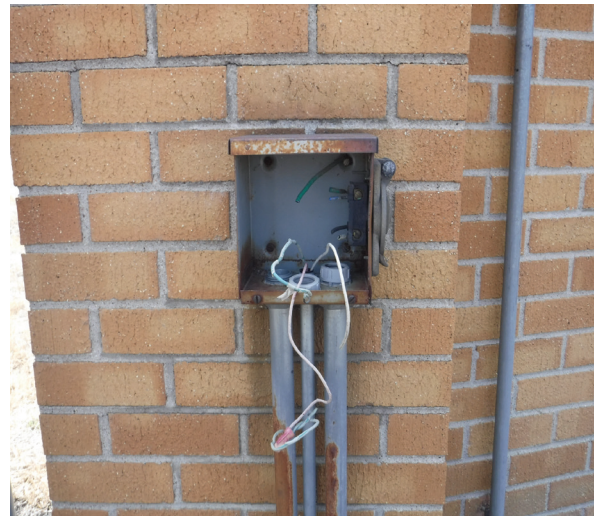
Unsafe/Exposed Electrical Wire
