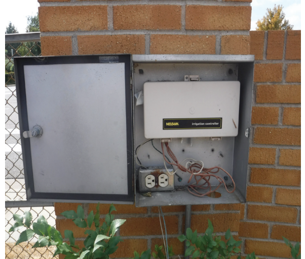
Unsafe/Exposed Electrical Wire
