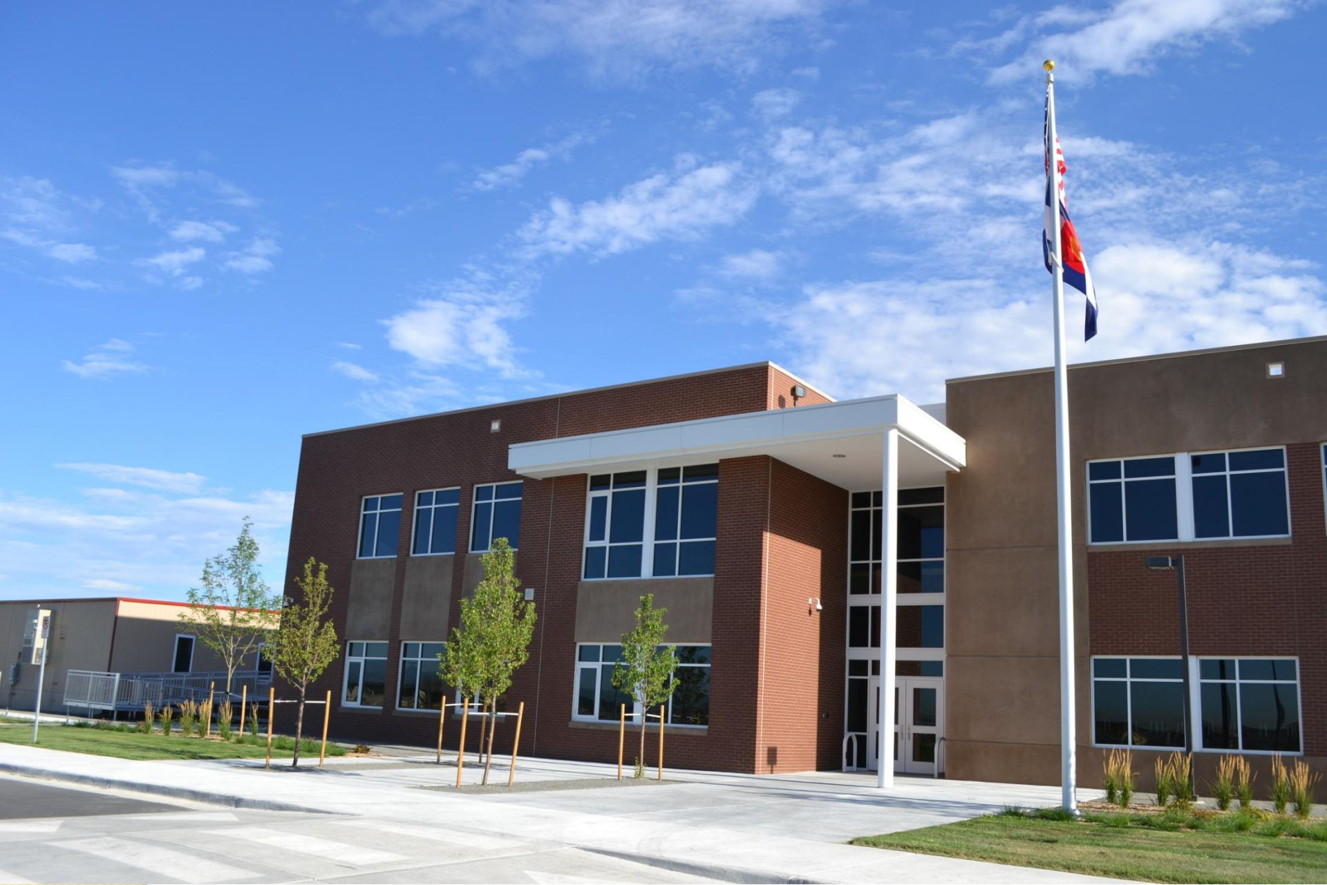
Brantner Elementary School Thornton
