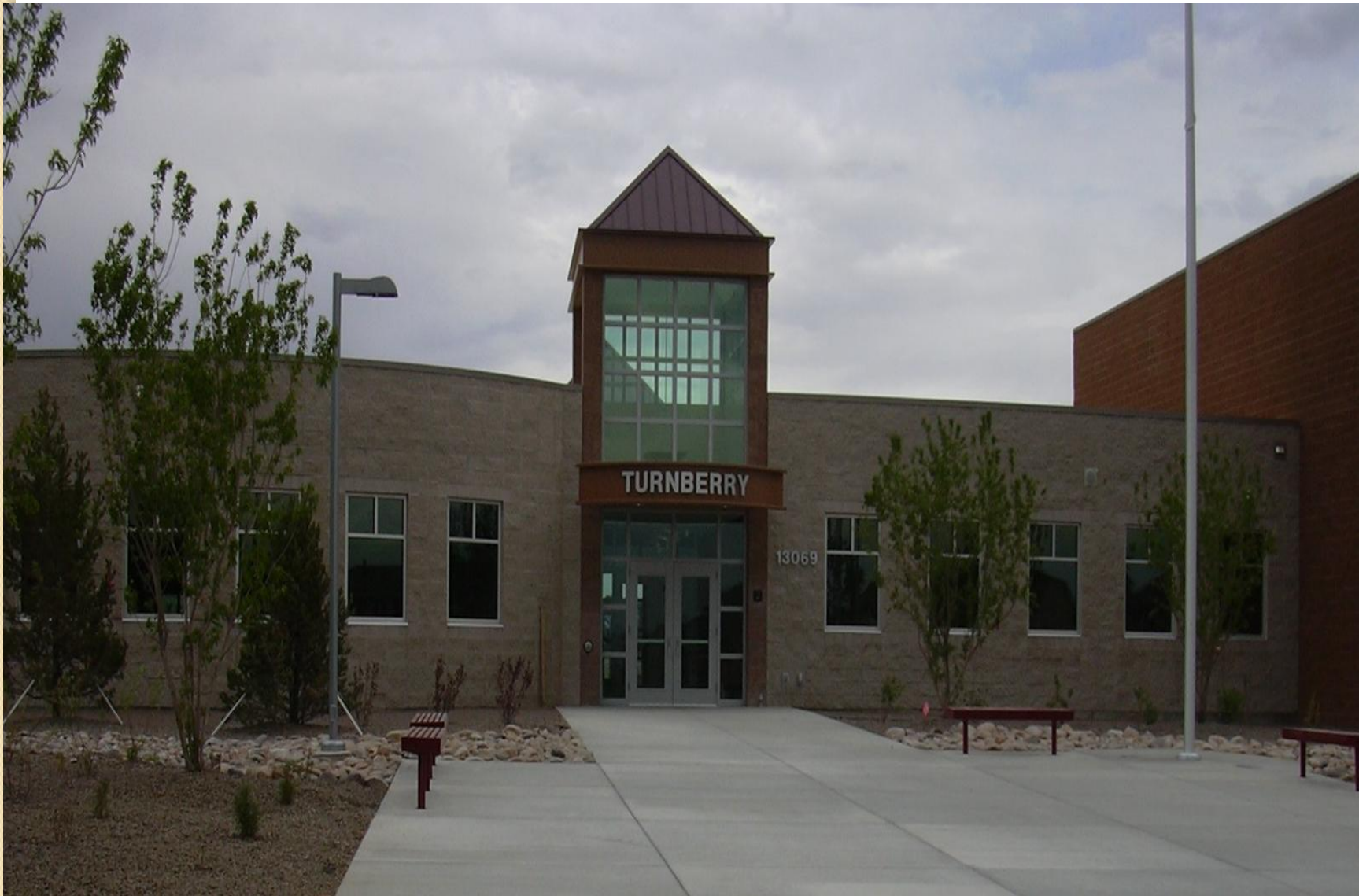
Turnberry Elementary School Commerce City
