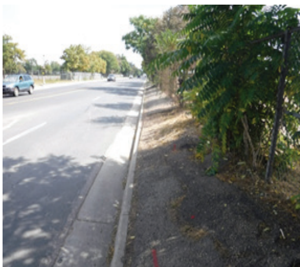
Lack of Sidewalk
