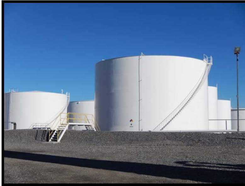
Figure 7: Fixed Cone Roof – Tank #6
