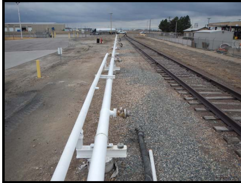
Figure 17: Existing Bottom-Unloading Location of Rail Cars
