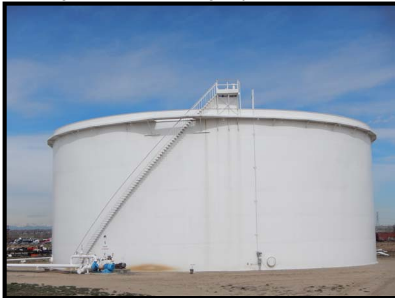
Figure 6: External Floating Roof – Tank #12
