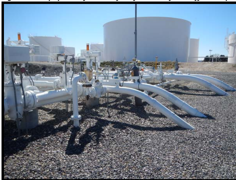
Figure 10: Equipment for Transfer of Product from Off-site Pipelines
