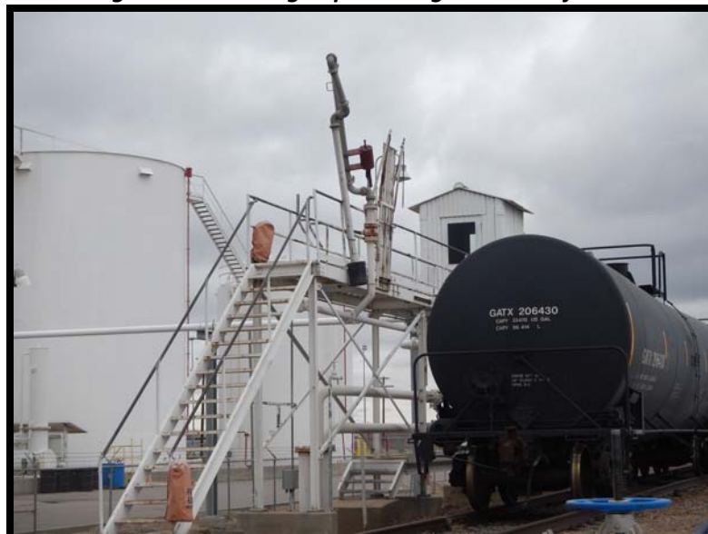
Figure 18: Existing Top-Loading Location of Rail Cars
