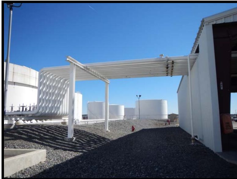
Figure 12: Equipment for Transfer of Product for and Between Truck Bays
