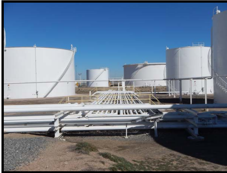
Figure 11: Equipment for Transfer of Product between Storage Tanks
