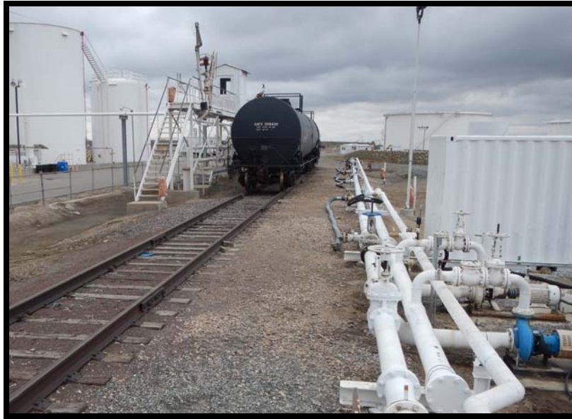
Figure 13: Equipment for Transfer of Product for Rail
