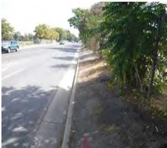
Lack of Sidewalk
