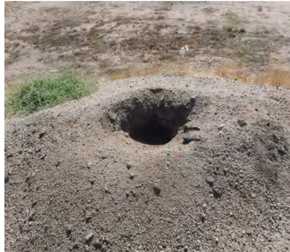
Evidence of Rodent Infestation
