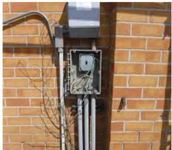
Exposed Wires
