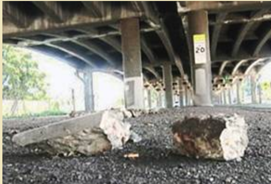
Falling pieces of concrete show a structurally deficient viaduct. The photo was taken on 46th Avenue under the viaduct.
