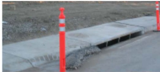
Properly installed inlet protection for continuous-grade curb-inlets.
