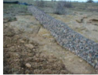
Reinforced rock berms are especially useful over bedrock outcroppings or pavement where silt fence and sediment control logs cannot be installed.
