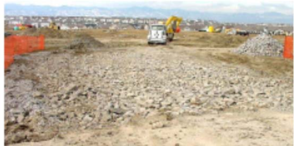
Properly installed vehicle tracking control.
