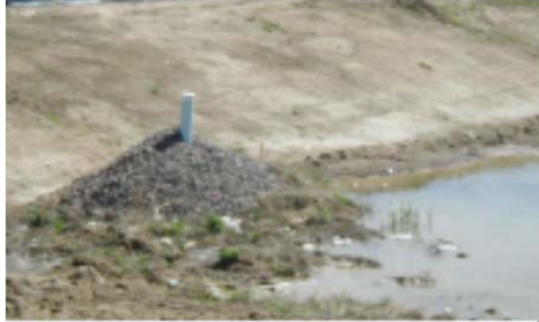
Properly installed outlet pipe and gravel pack.
