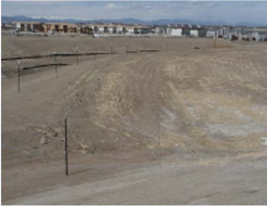
This diversion ditch provides protection for an adjacent drainageway.
