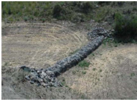
Reinforced check dams are required in major drainageways to resist breaching from overtopping flows.
