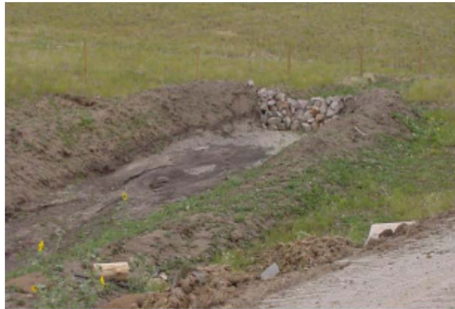
A properly installed sediment trap.
