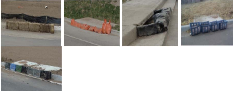
Blocking the inlet opening or use of alternate materials for inlet protection is prohibited.
