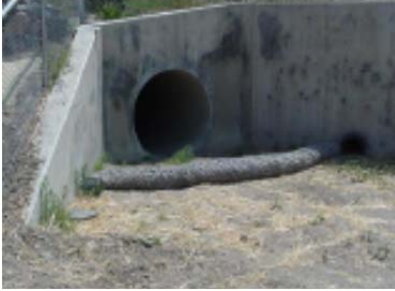
A properly installed reinforced rock berm for culvert protection.
