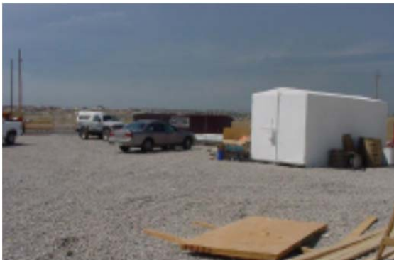
Properly installed stabilized staging area.
