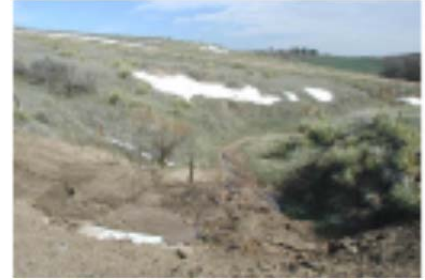
This disturbed drainageway was not protected by a check dam at the downstream site perimeter, allowing sediment to be conveyed off site.
