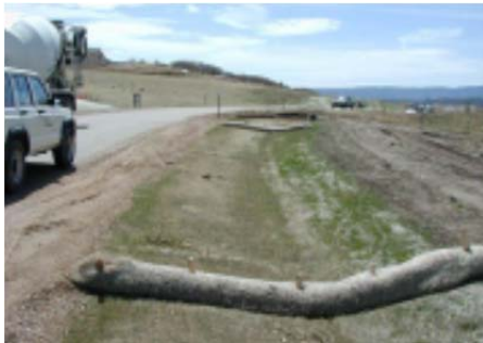
Sediment control logs shall not be installed in roadside ditches or other concentrated flow areas.
