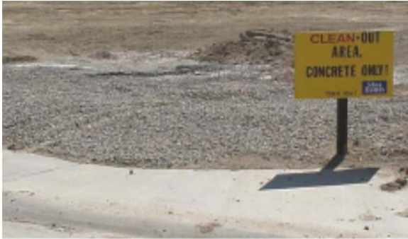
A properly installed concrete washout area with Vehicle Tracking Control.
