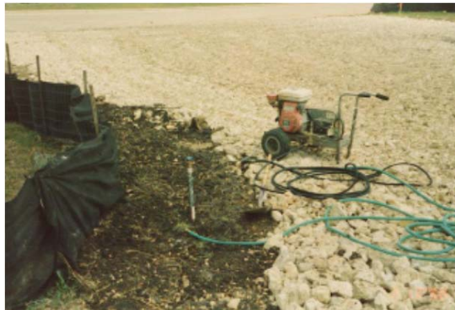
A high-pressure washer effectively cleans mud from wheels.
