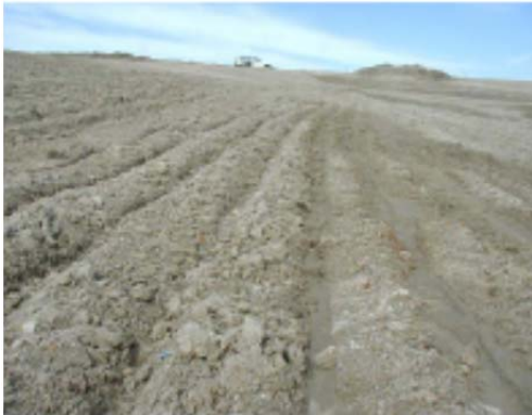
Properly executed surfacing roughening.
