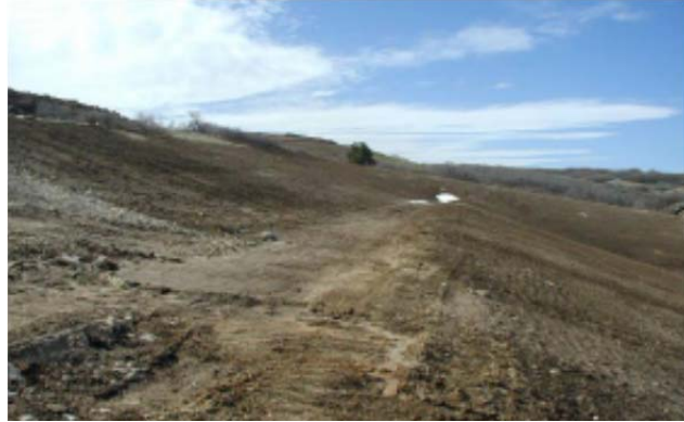
This terraced bench interrupts slope drainage and reduces rill and gully erosion.
