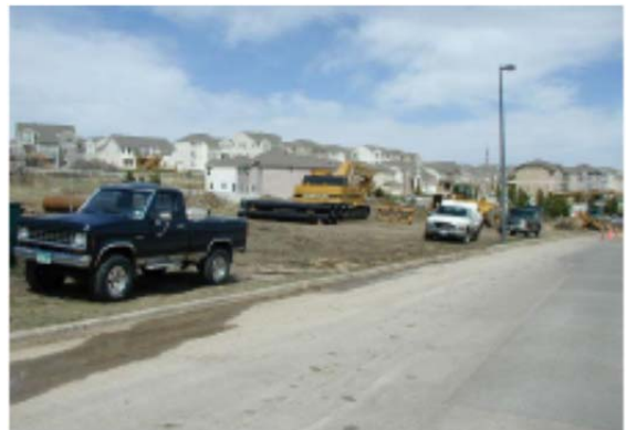
Parking, staging, and storage are spread out all over this site, increasing disturbance and erosion.
