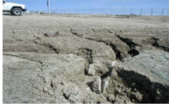
Lack of a diversion ditch at the top of this slope to divert upstream runoff has led to severe rill and gully erosion.
