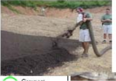
Compost blankets can be used in areas not subject to concentrated flows and shall be applied with a pneumatic blower or by hand.
