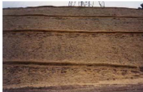
Sediment control logs shall not be installed in roadside ditches or other concentrated flow areas.
