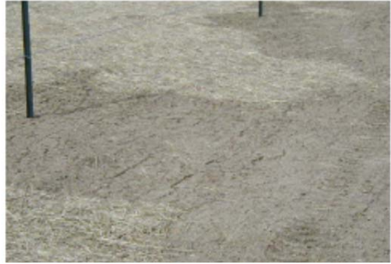
This mulch was not crimped into soil and is susceptible to displacement, leaving the seed bed unprotected.
