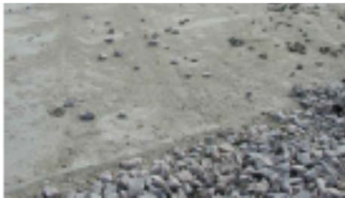
Use of low density rock such as Rhyolite is not permitted since it does not stay in place and can get tracked onto paved streets.
