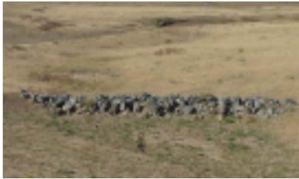
Properly installed check dam.
