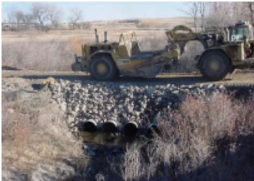
Properly installed temporary stream crossing.
