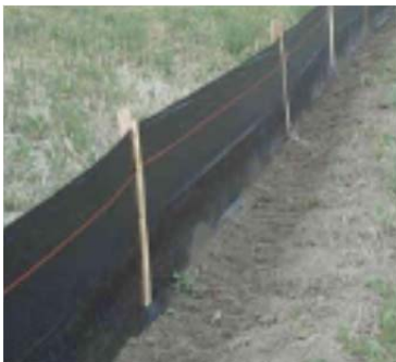
Properly installed silt fence cannot easily be pulled out of the ground.
