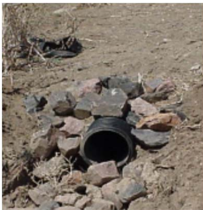
Properly installed temporary slope drain pipe alternative).
