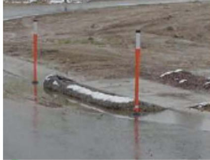
Properly installed inlet protection for curb-inlets in a sump condition.
