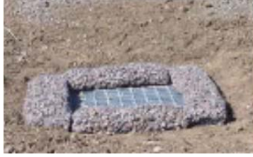
Properly installed area inlet protection.
