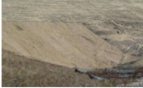
Ample erosion control blanket is used on this hill slope.
