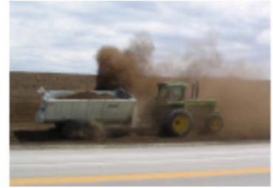
Utilizing non-approved application methods of compost blanket can cause additional cost due to re-application and additional clean up costs.
