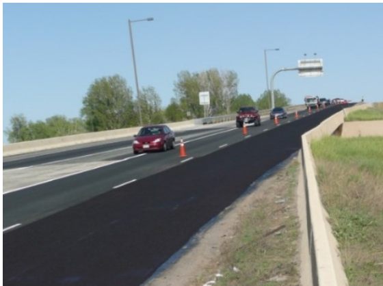
Micro surfacing Application
