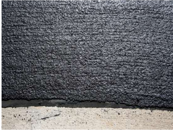
Slurry Seal Application
