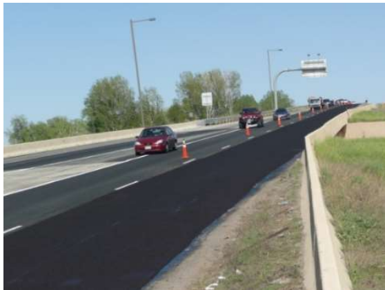
Micro surfacing Application
