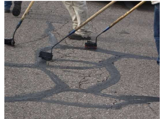
Crack Sealing/Filling
