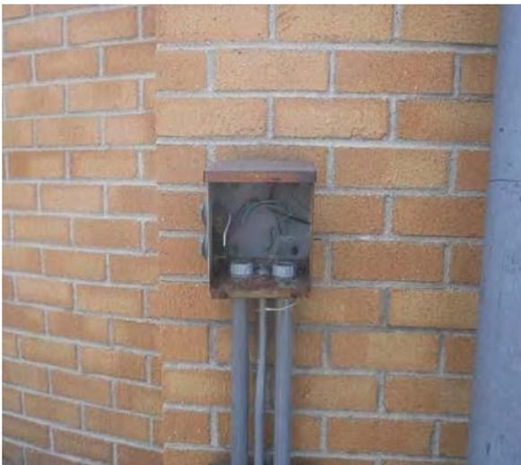
Unsafe/Exposed Electrical Wire
