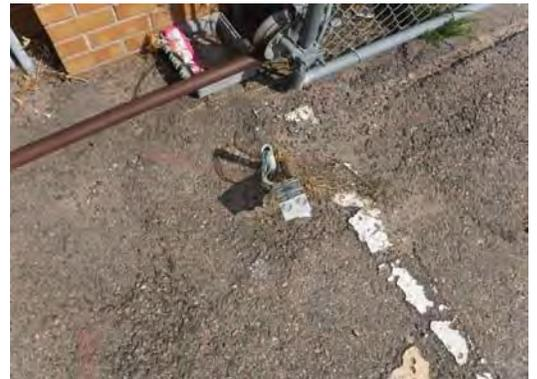
Unsafe/Exposed Electrical Wire
