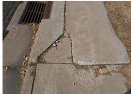
Cracked/Uneven Pedestrian Surfaces
