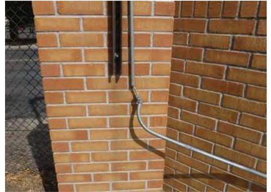
Unsafe/Exposed Electrical Wire
