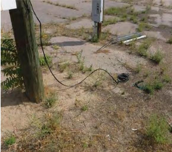
Unsafe/Exposed Electrical Wire
