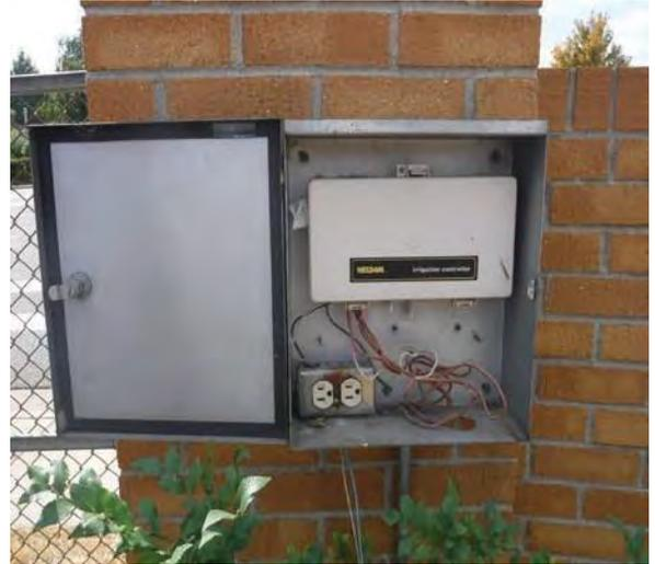
Unsafe/Exposed Electrical Wire
