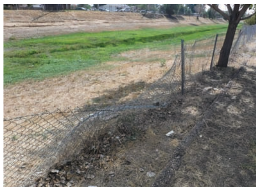
Dilapidated/Deteriorated Fencing
