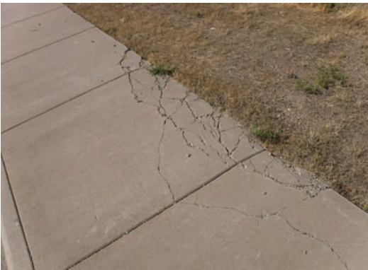
Deteriorated Curb/Sidewalk
