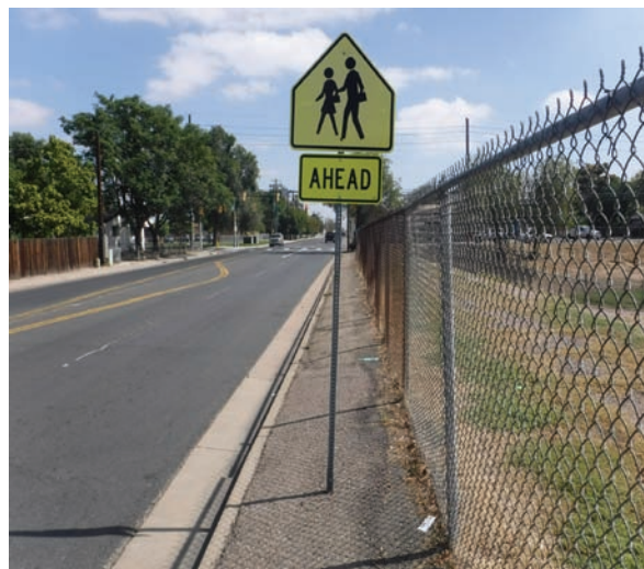
Pedestrian Barrier Resulting in Vehicle Conflict
