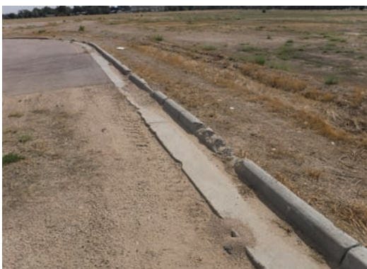
Deteriorated Curb/Sidewalk
