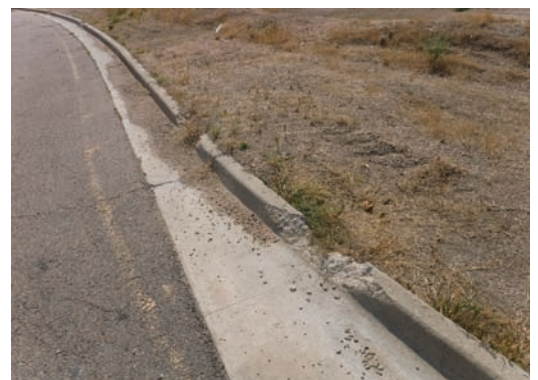
Deteriorated Curb/Sidewalk
