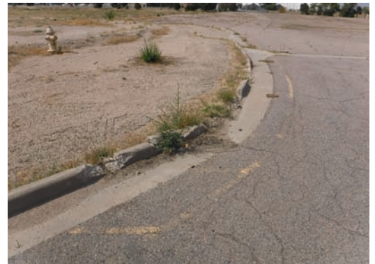
Deteriorated Curb/Sidewalk
