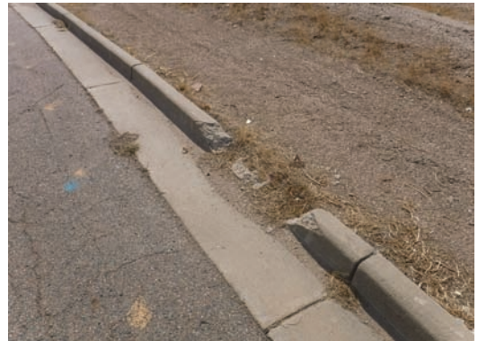
Deteriorated Curb/Sidewalk
