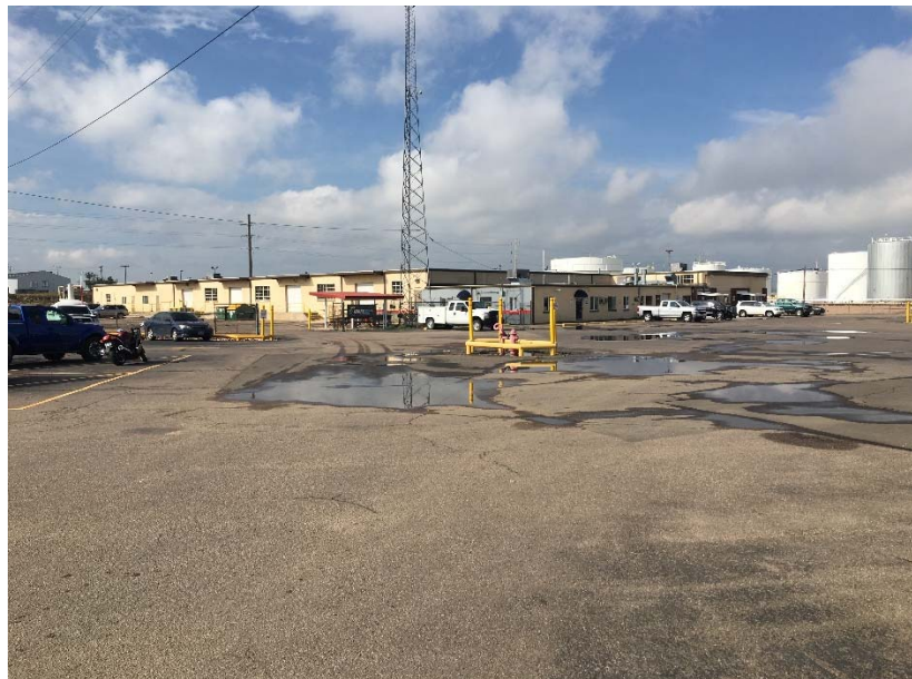
Administrative office/Warehouse building
