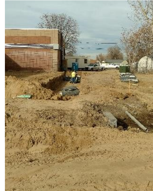
Foundation Excavation
