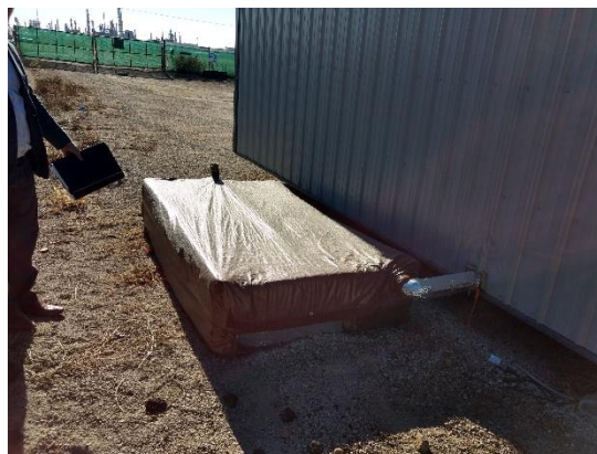
ABOVE GROUND SEPTIC TANK REMOVED
