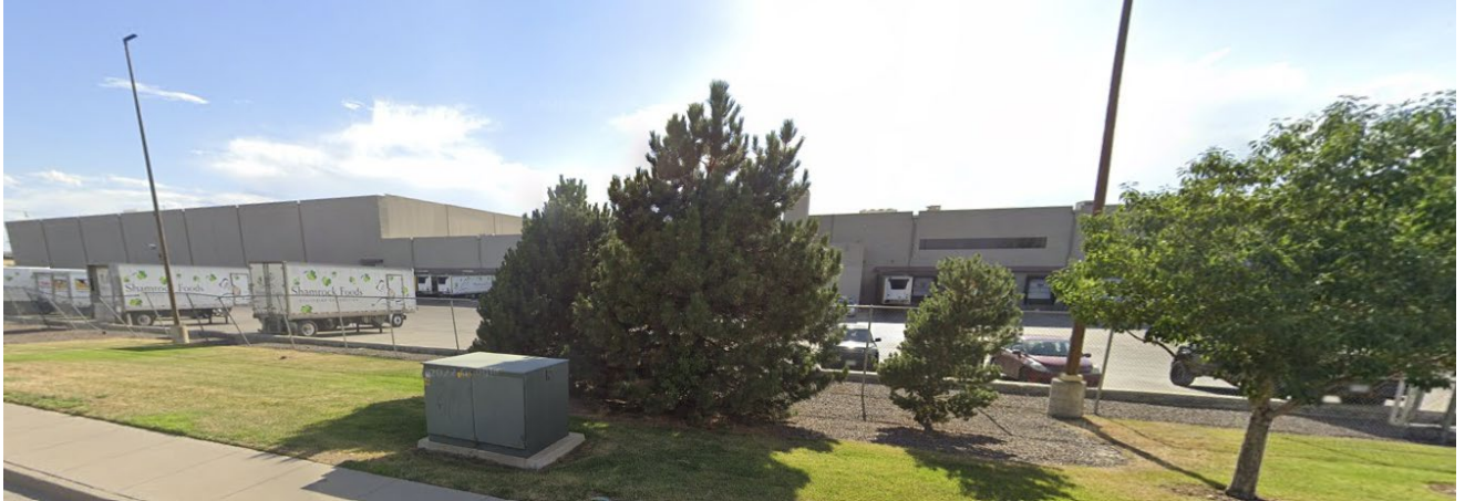
Transportation Terminal facing west from Ivy Street
