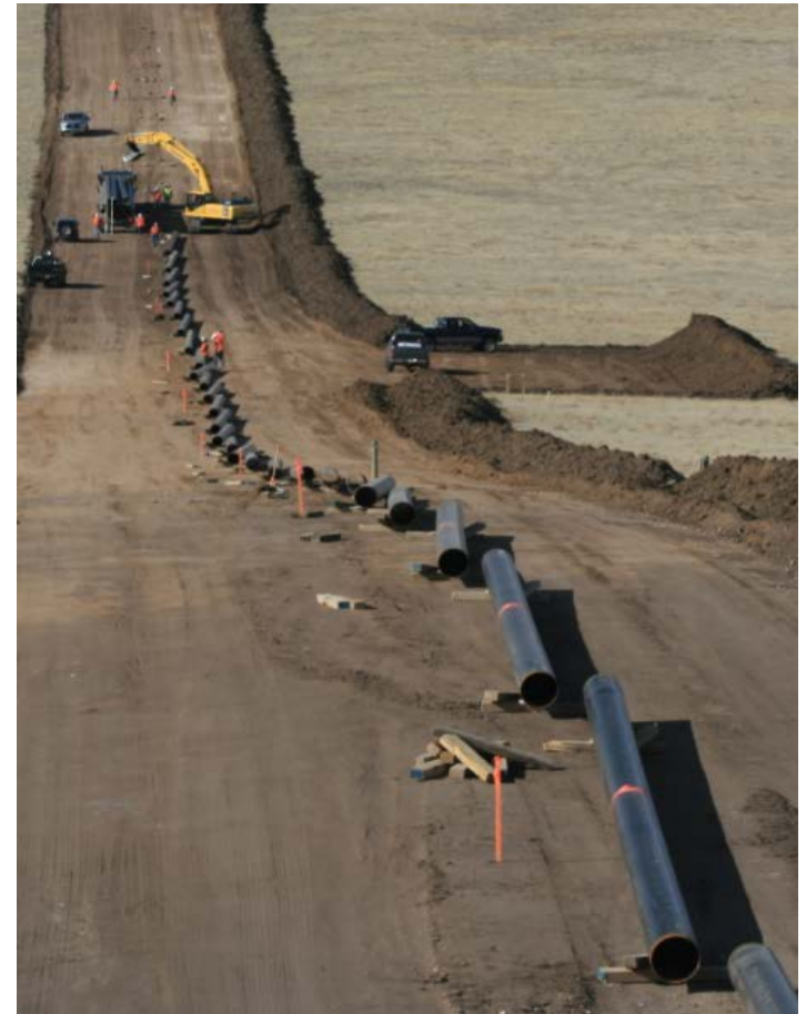
Stringing the pipe
