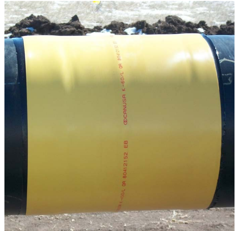
Coated girth weld
