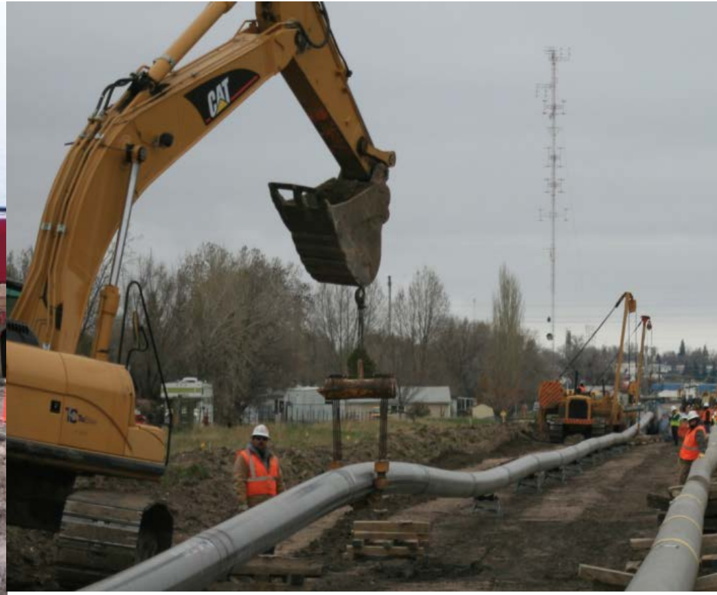
HDD pipe string ready for pullback
