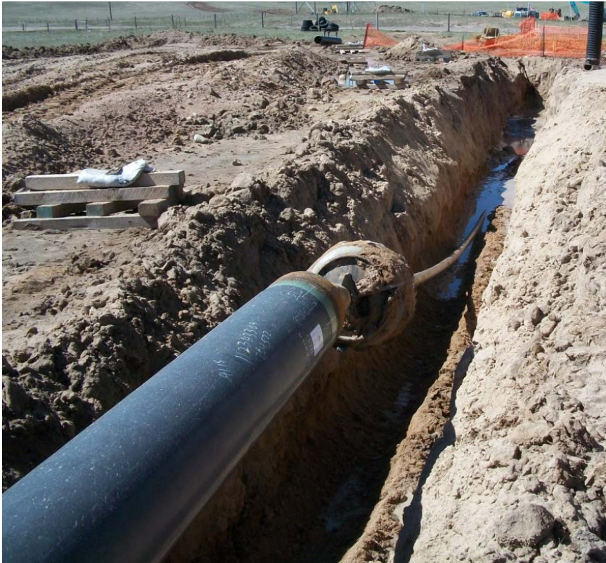
Pipe attached to pull head
