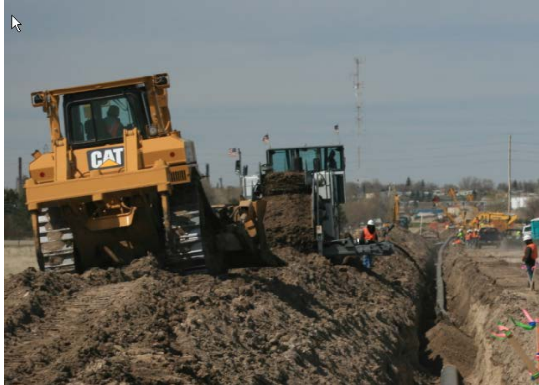
Starting to pad & backfill
