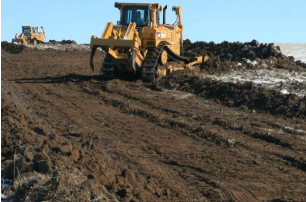
Clearing/grading the R/W
