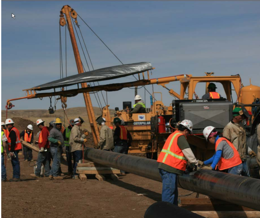
Pipe line-up & welding
