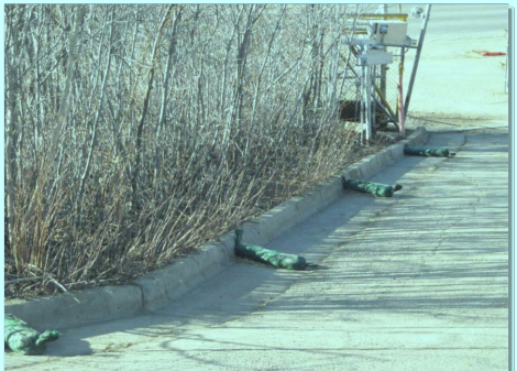
Photograph RS-1: Rock socks placed at regular intervals in a curb line to help reduce sediment loading to storm sewer inlets. Rock socks can also be used as perimeter controls.
