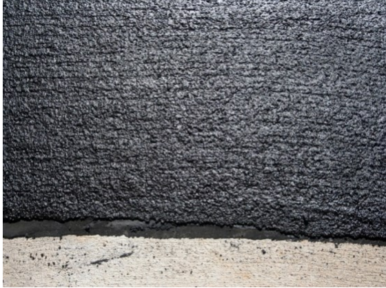
Slurry Seal Application
