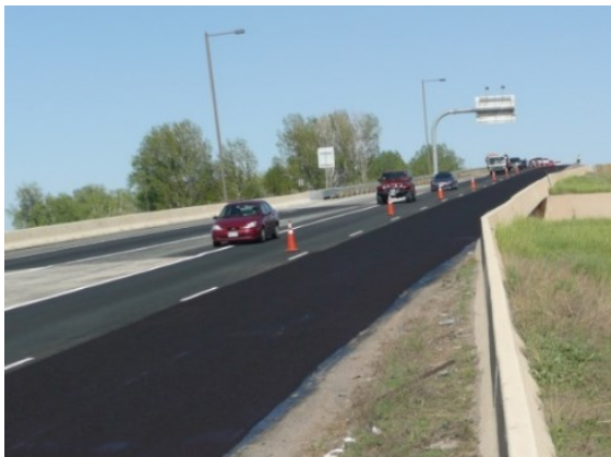
Micro surfacing Application
