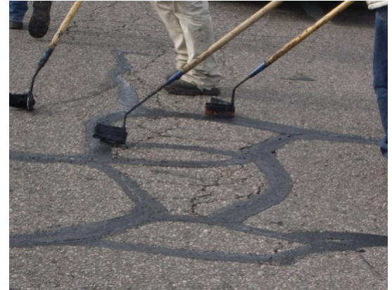
Crack Sealing/Filling
